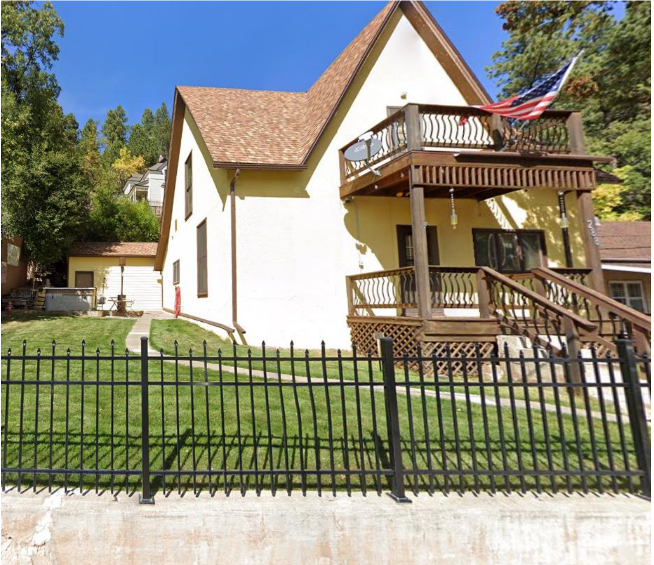
Photo showing current garage configuration at 288 Williams Street.
