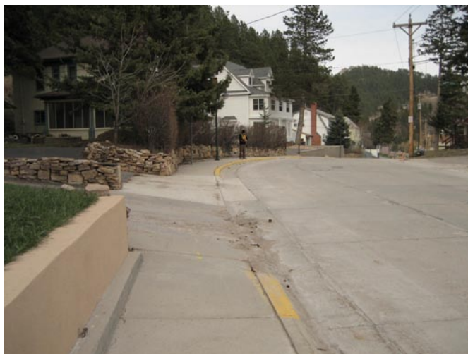
Cross-slope across driveways is a common deficiency for Deadwood sidewalks. A 36 inch wide sidewalk travel way in combination with a compound apron slope can often mitigate this type of cross slope deficiency (see sketches).
