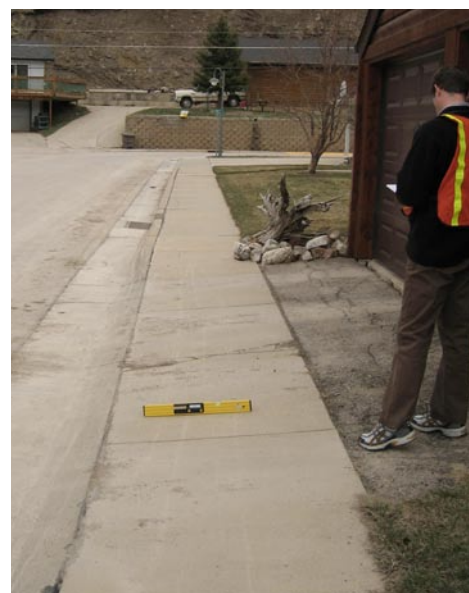
A field inventory of sidewalks included sidewalk termini, width, curb height, cross-slope, surface material, horizontal and vertical cracks, in-sidewalk obstructions, and curb ramps.
