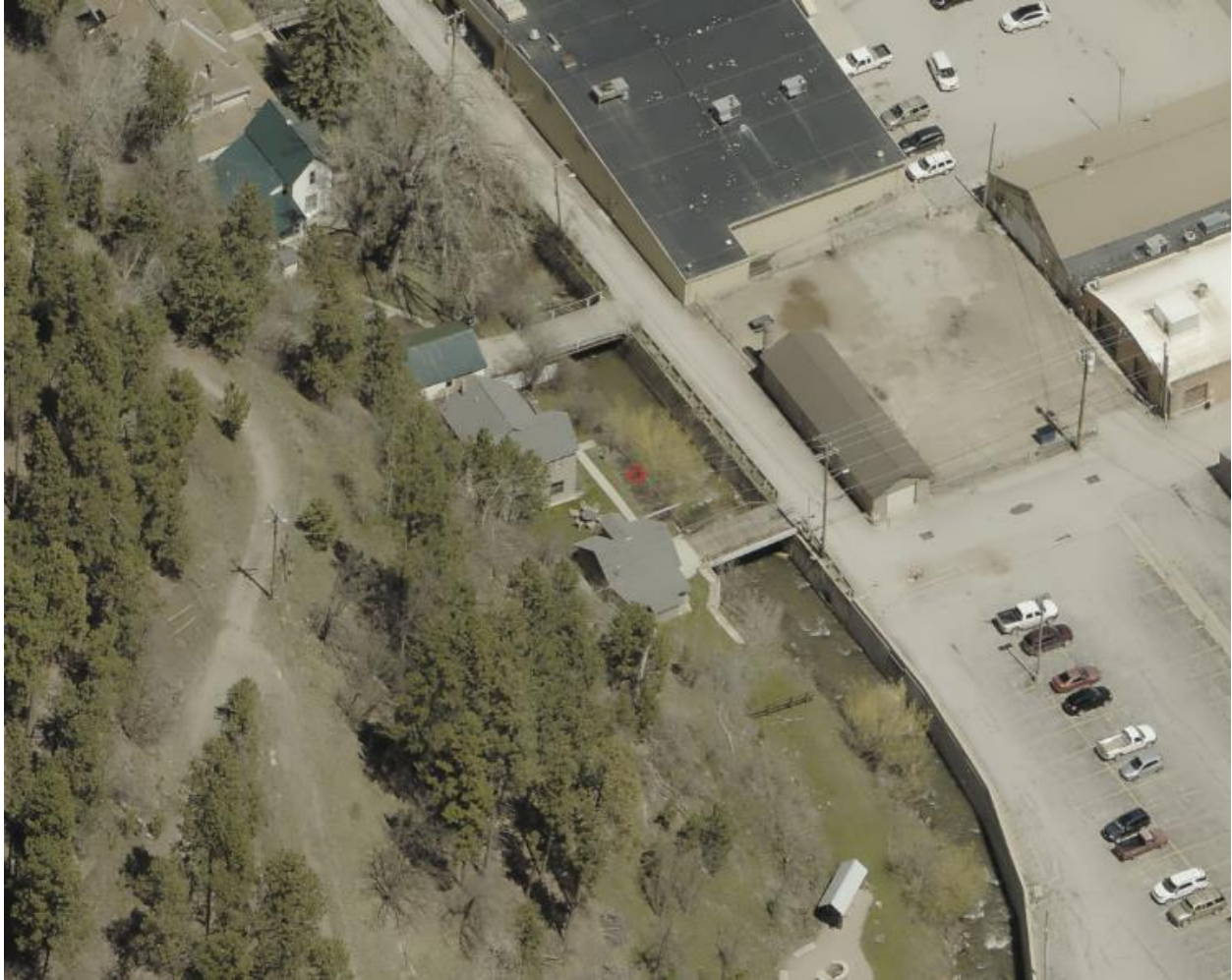
Aerial view of 36 Water Street.
