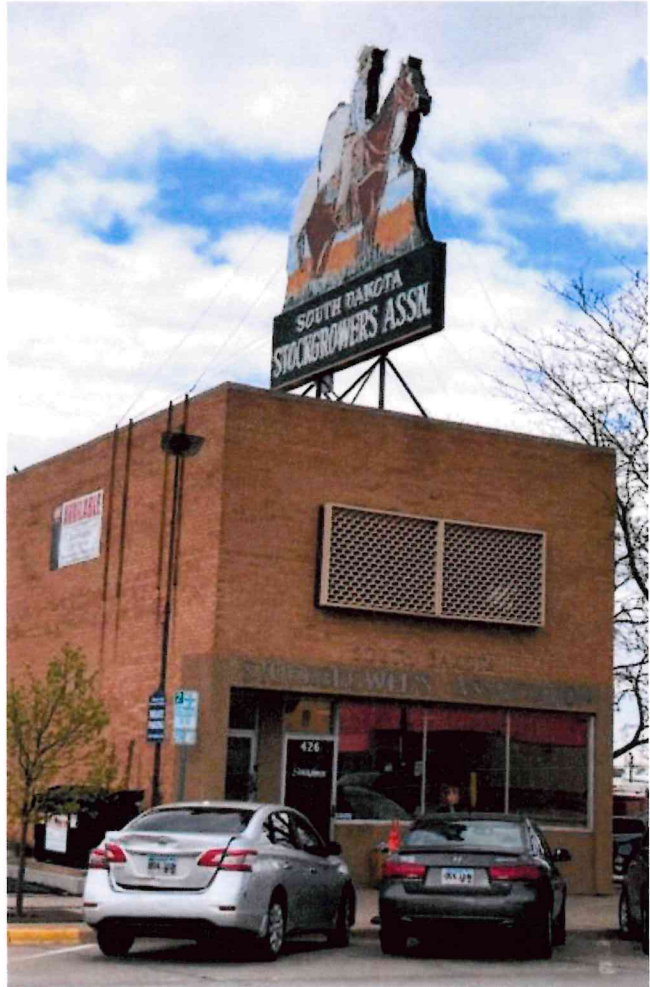
The South Dakota Stockgrowers Association building has been part of downtown Rapid City since it was constructed in the 1950s.
