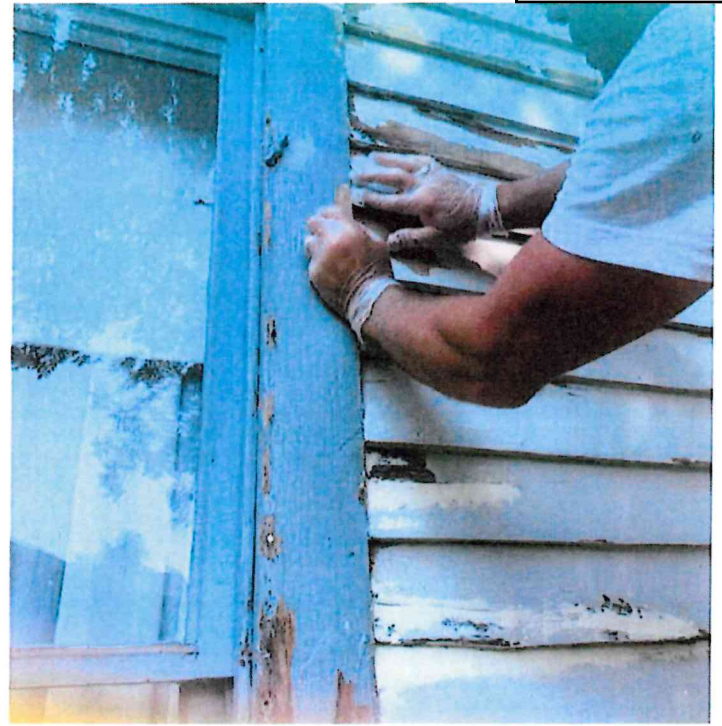
Contractor at work on the West side of the building
