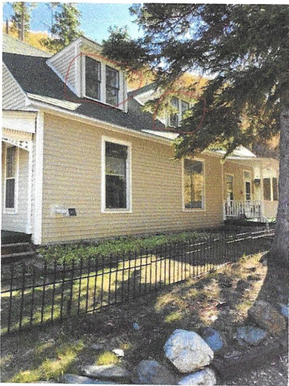
This is the right side of the house. The four windows circled in red in the upper two dormers need to be replaced.
