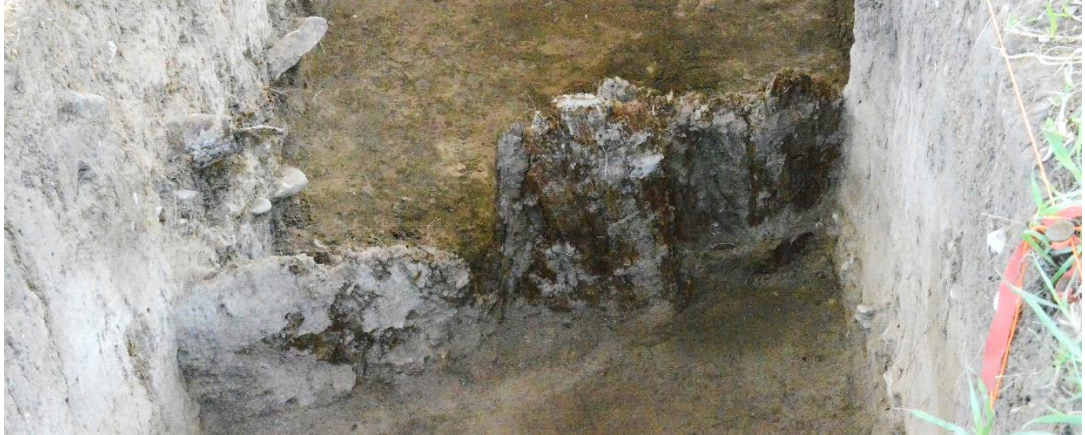
Figure 17. Side view of plank wall at termination of excavation, facing south
