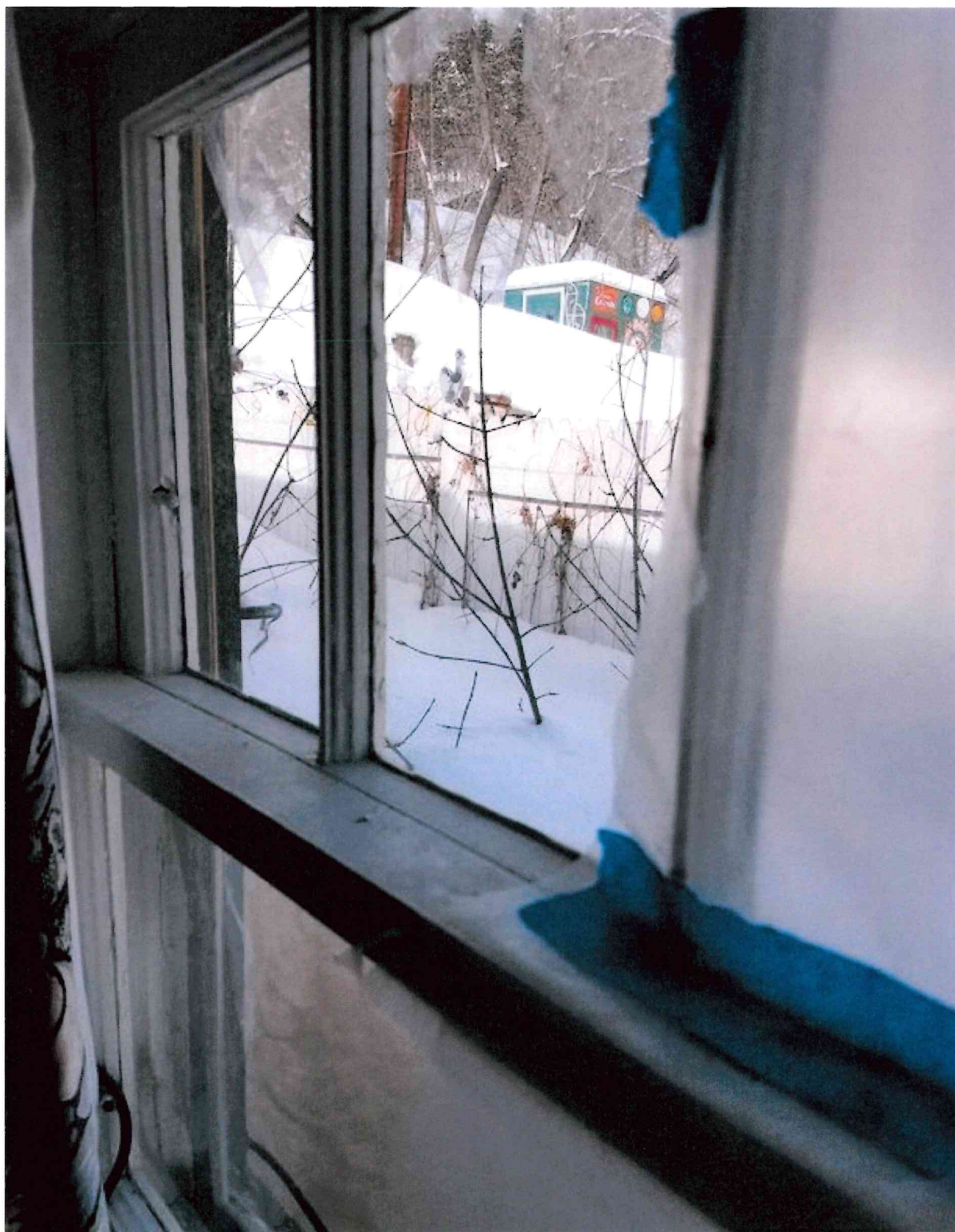
Inside Kitchen Windows – Broken and painted shut
