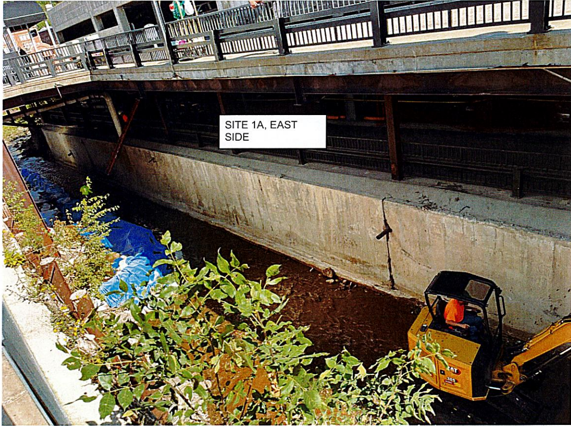
NOTE: AREA JUST DOWNSTREAM FROM PHOTO ON PAGE 3.
