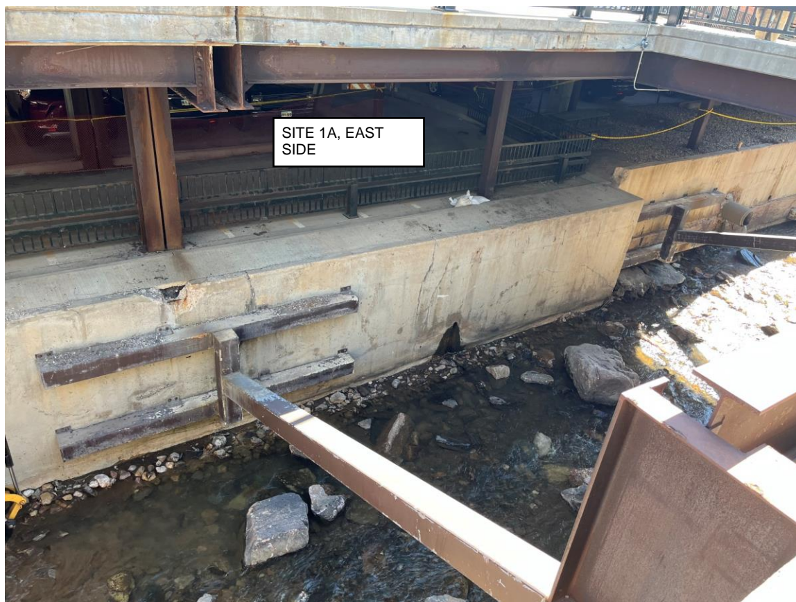
NOTE: AREA JUST UPSTREAM FROM PHOTO ON PAGE 3.
