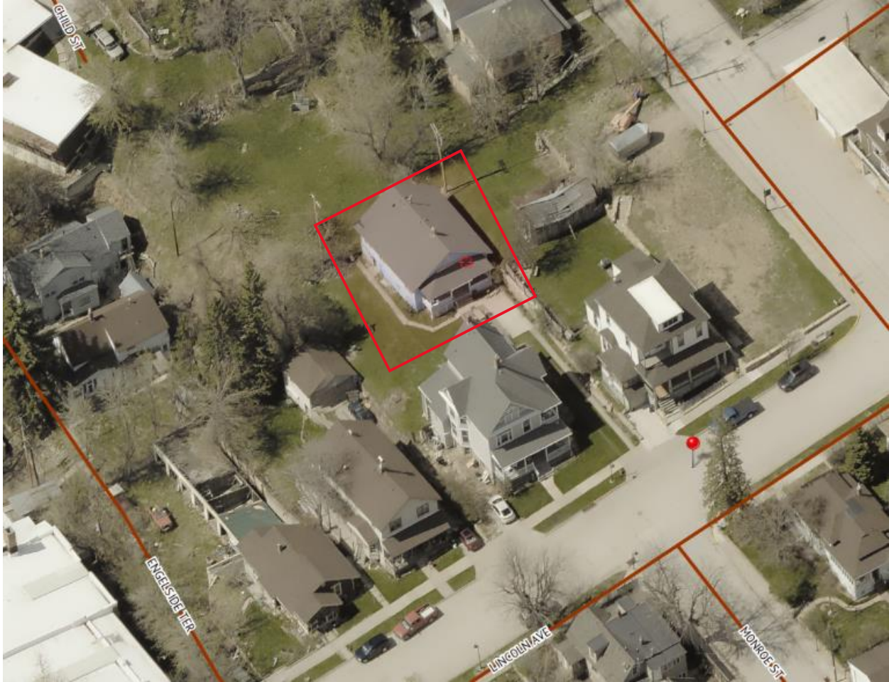
Aerial view of 25 Lincoln Ave, Deadwood, SD 57732.
