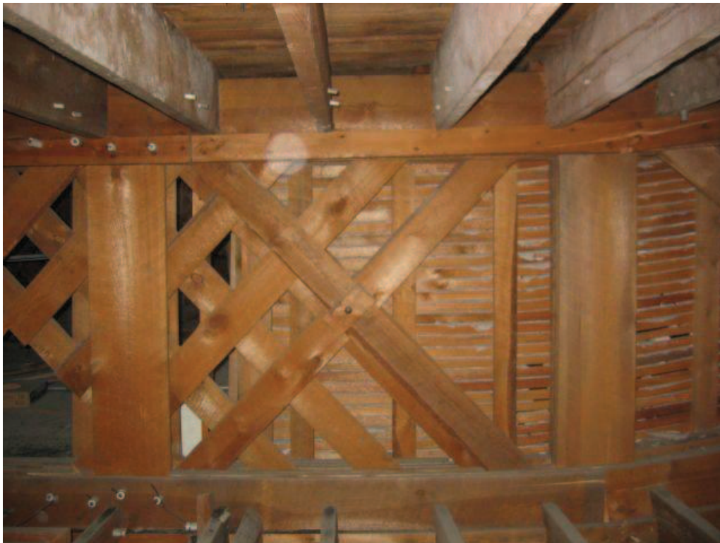
Photo No. 24: Interior panel of subject girder truss. View is at the north end, looking to the west.
