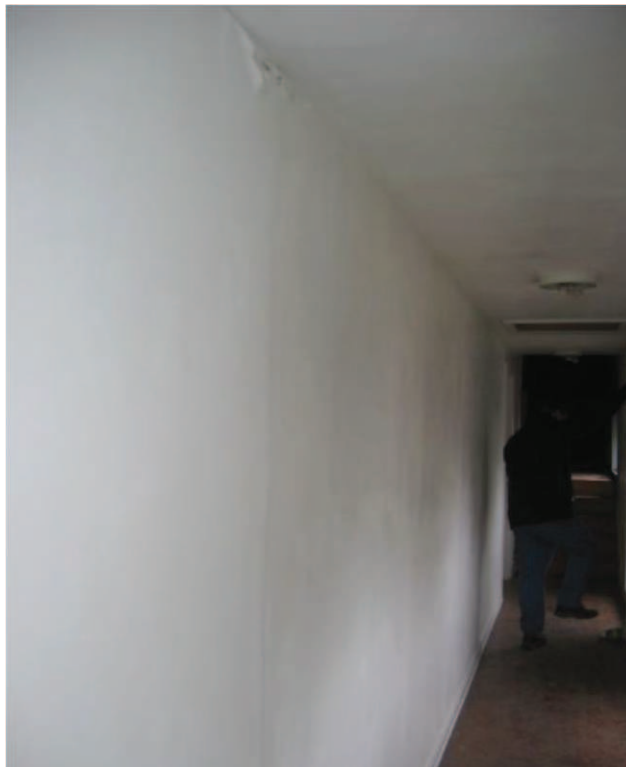
Photo No. 6: Corridor along south side of building at girder truss bearing.
