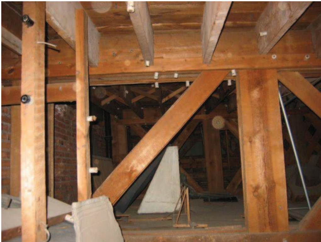
Photo No. 30: South end of subject girder truss.
