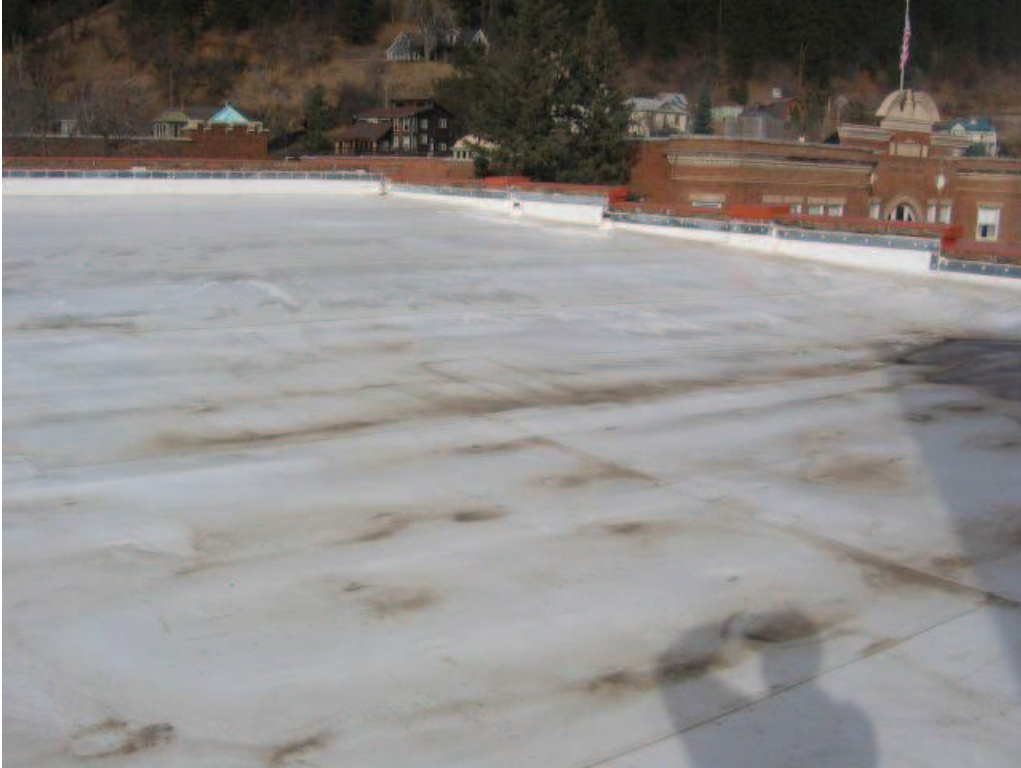
Photo No. 35: North parapet wall, west end.
