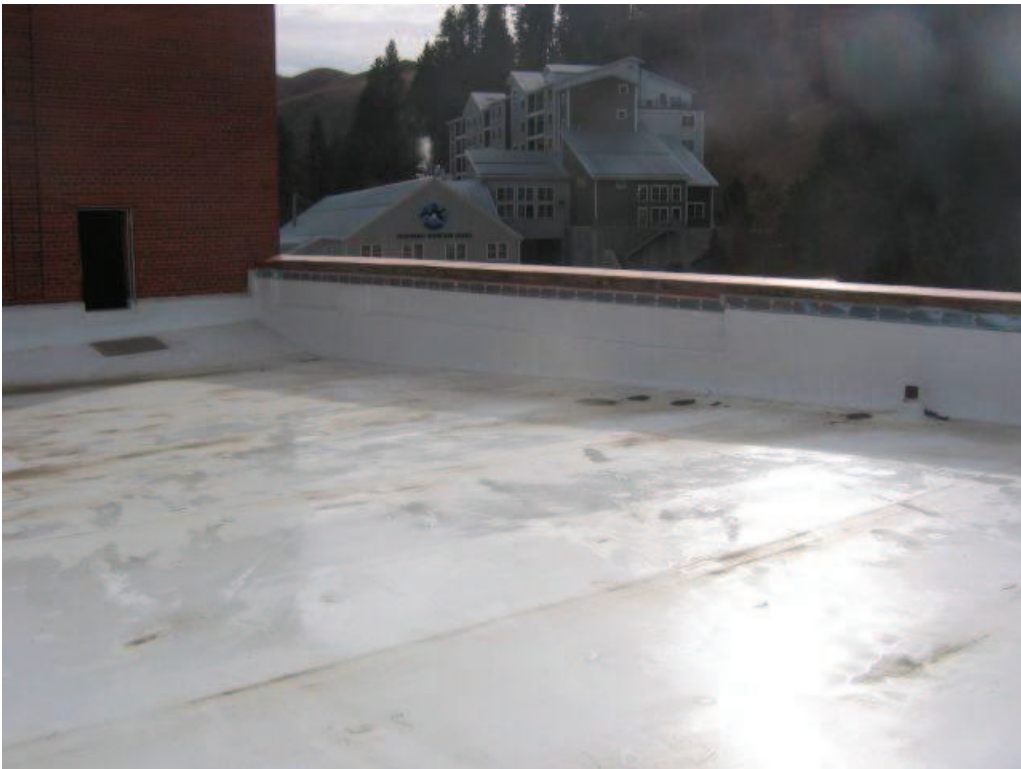
Photo No. 36: Southeast parapet wall, approximately 55-inches high.
