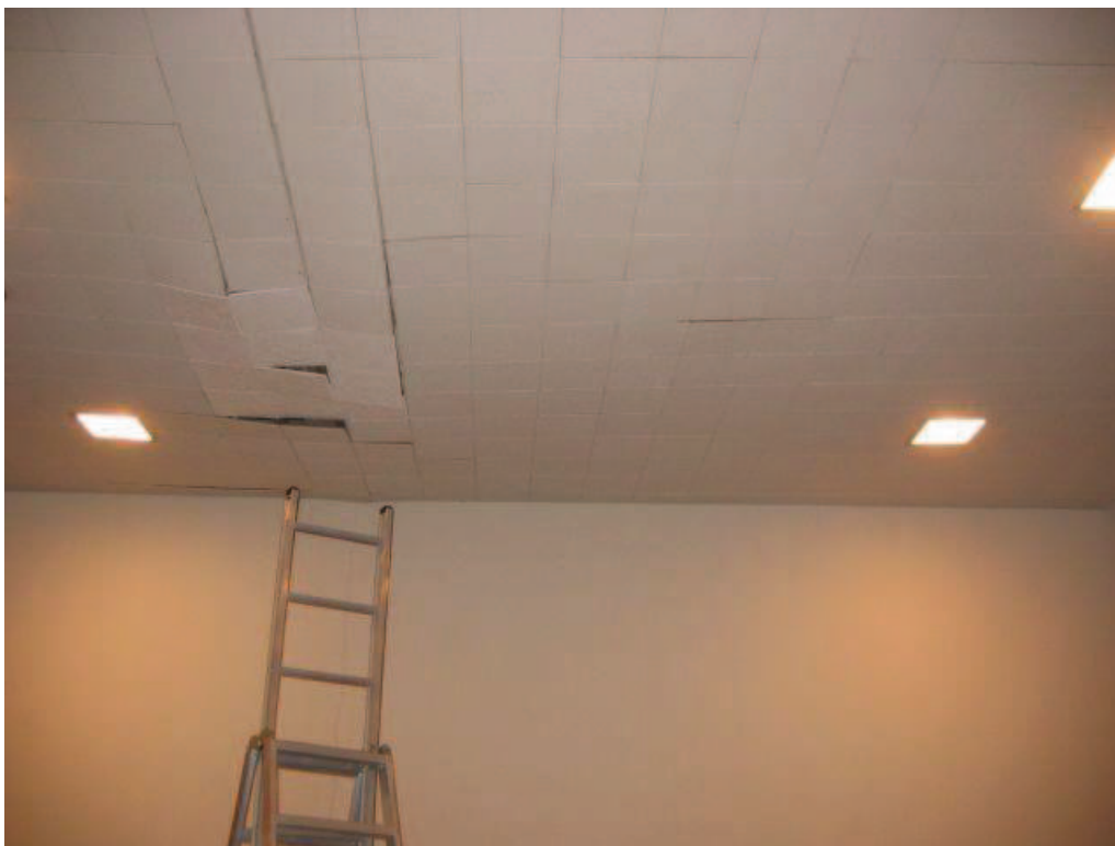
Photo No. 2: Displaced ceiling tile in auditorium at north end of girder truss.
