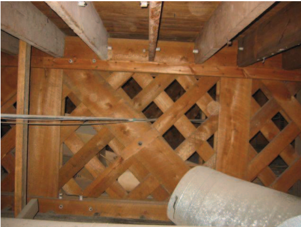
Photo No. 26: Interior panel of subject girder truss.
