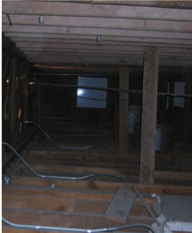
Photo No. 23: Typical ceiling and roof framing on east side of subject girder truss.
