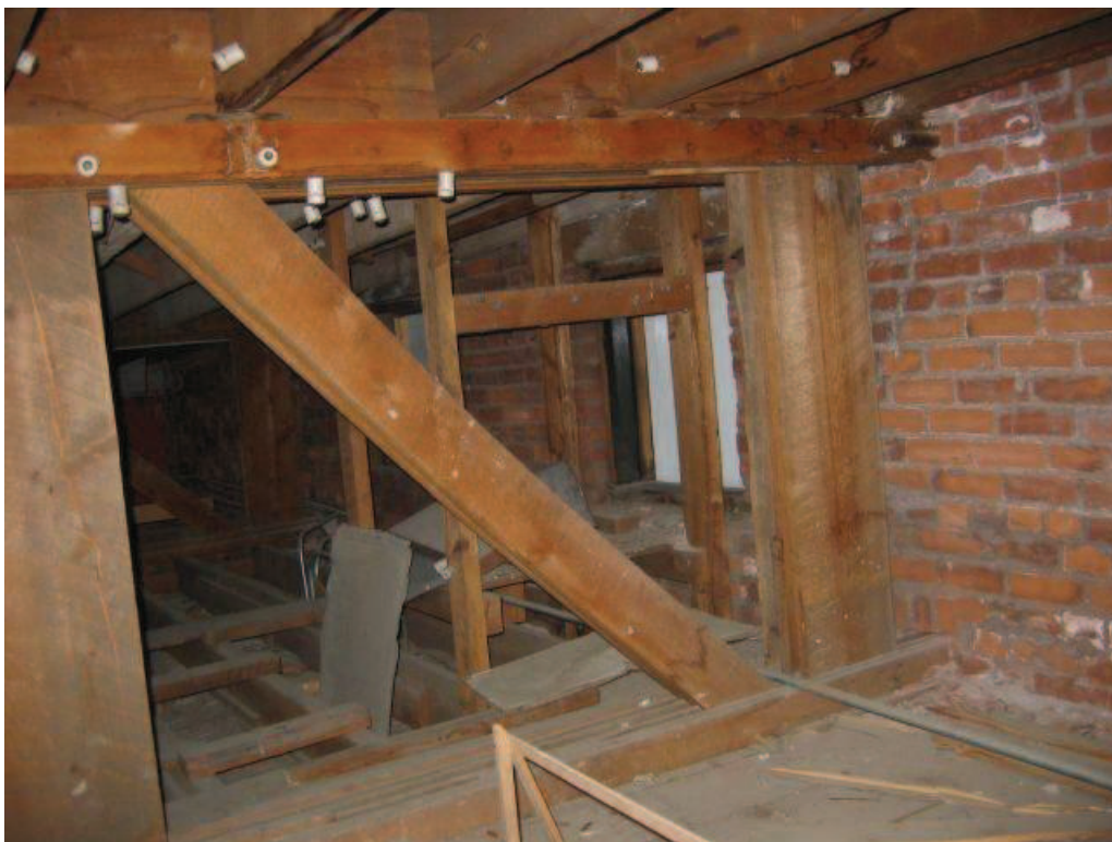
Photo No. 18: South end of girder truss, bearing point on brick wall.
