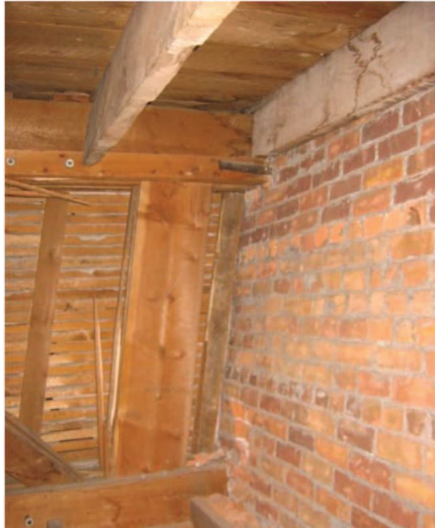
Photo No. 13: North end of girder truss, bearing at brick wall.
