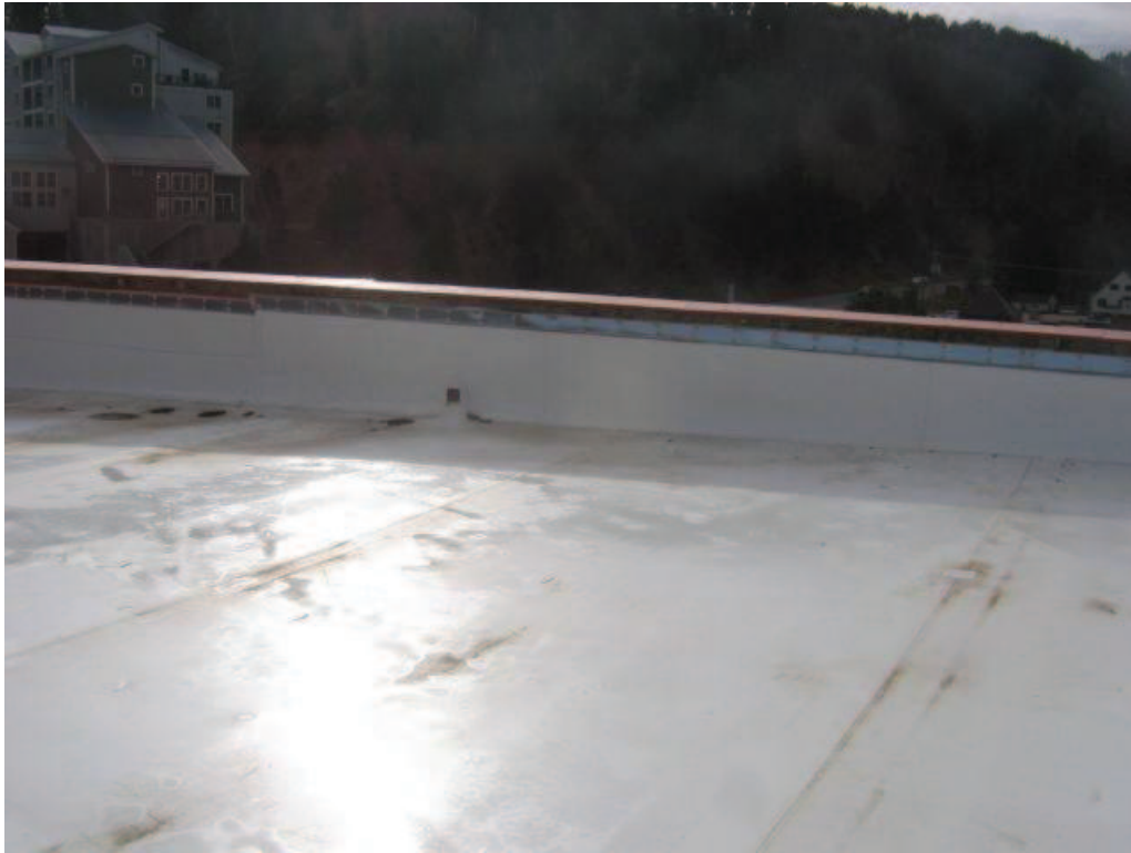
Photo No. 37: South parapet wall.
