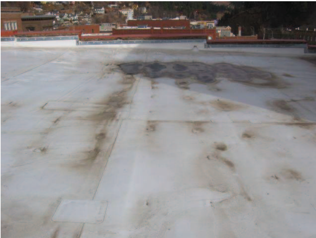
Photo No. 40: North end of truss deflected downward.
