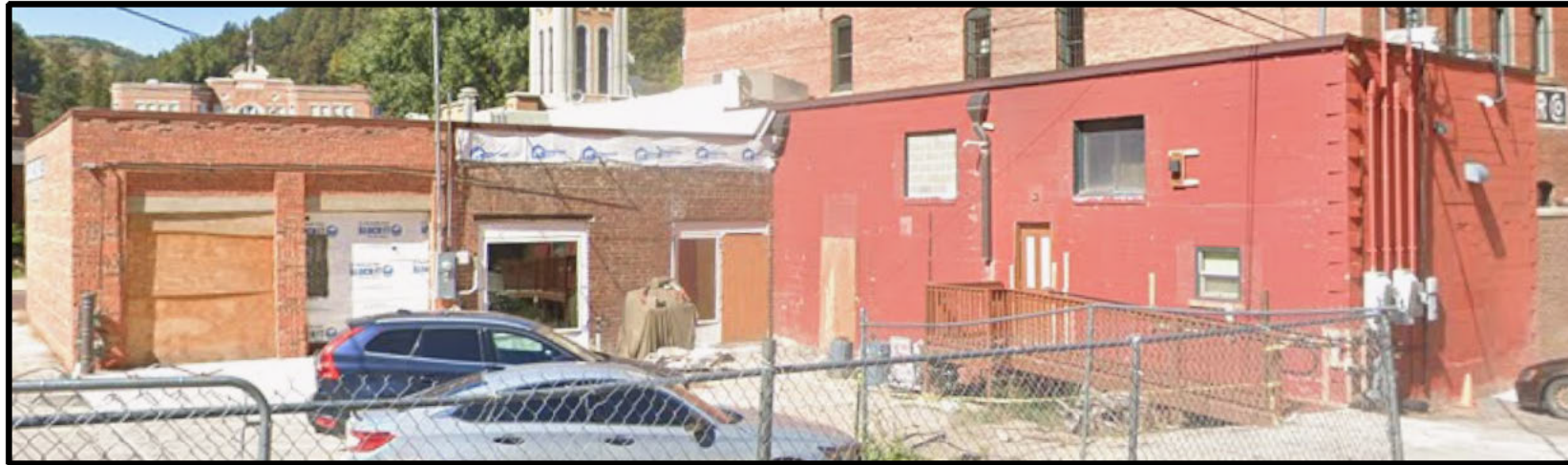
EXISTING SITE CONDITIONS
