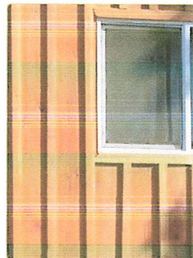
EXTERIOR SIDING : DOUGLAS FIR: ROUGH CUT Douglas Fir Board and batton detail of exterior siding installation.
