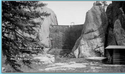
Sylvan Lake Dam (undated)
