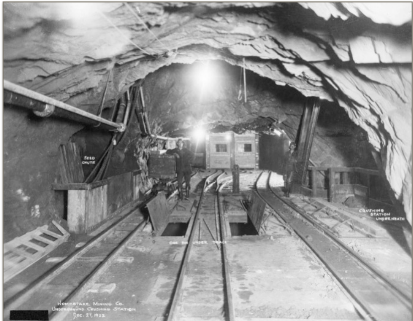
Underground crushing station, 1922.
