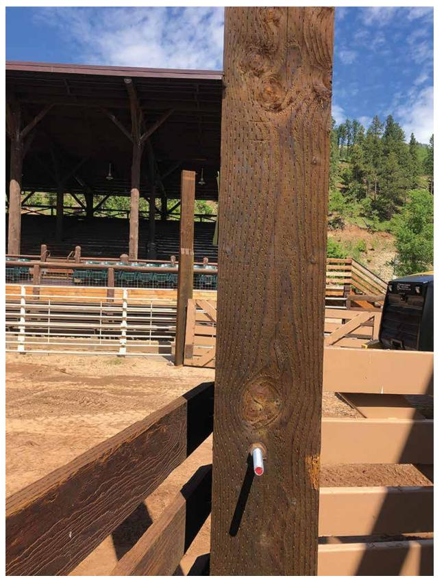
IMAGE SHOW THE 3'-6"+/- OFFSET OF THE POSTS AND THAT POST RETURNS/FACES ARE NOT PARALLEL TO ONE ANOTHER.
