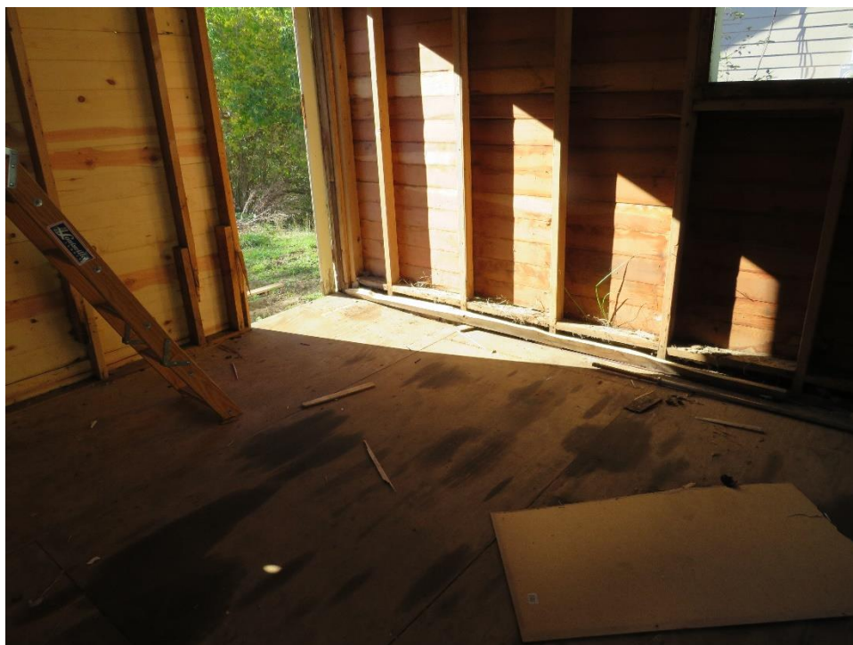
This photograph shows the two separate bottom plates and a bow in the floor.
