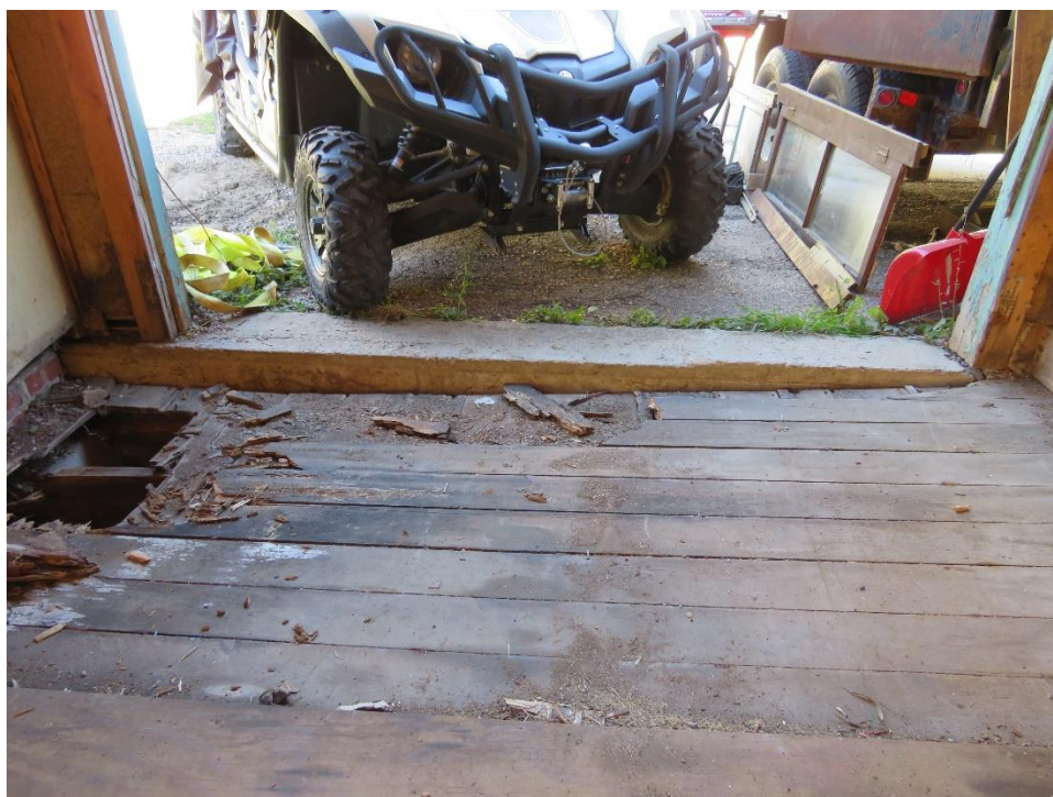
Photograph showing the area of the floor opened up by the applicant verifying construction method and deteriorated conditions.
