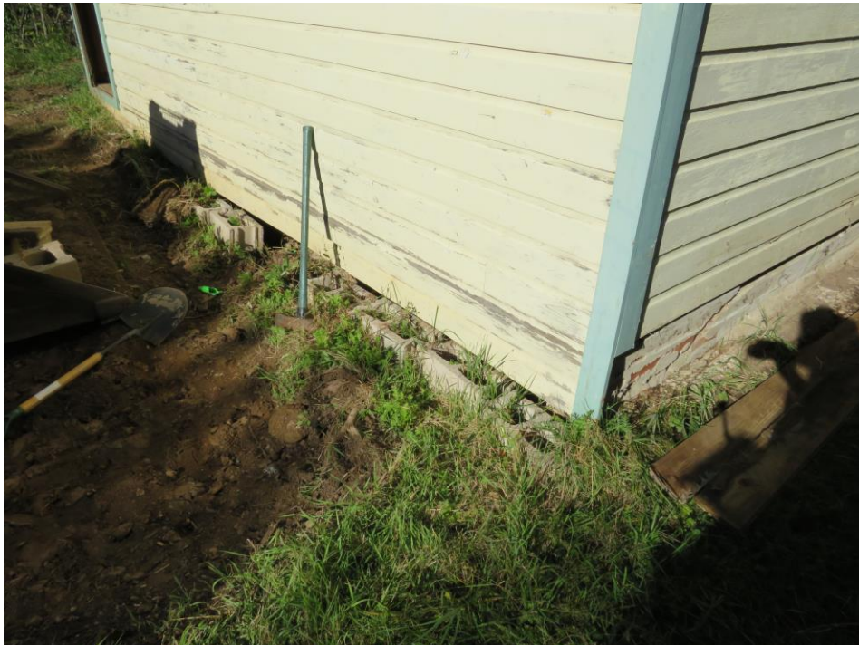
These photographs show the back side of the structure off the foundation.
