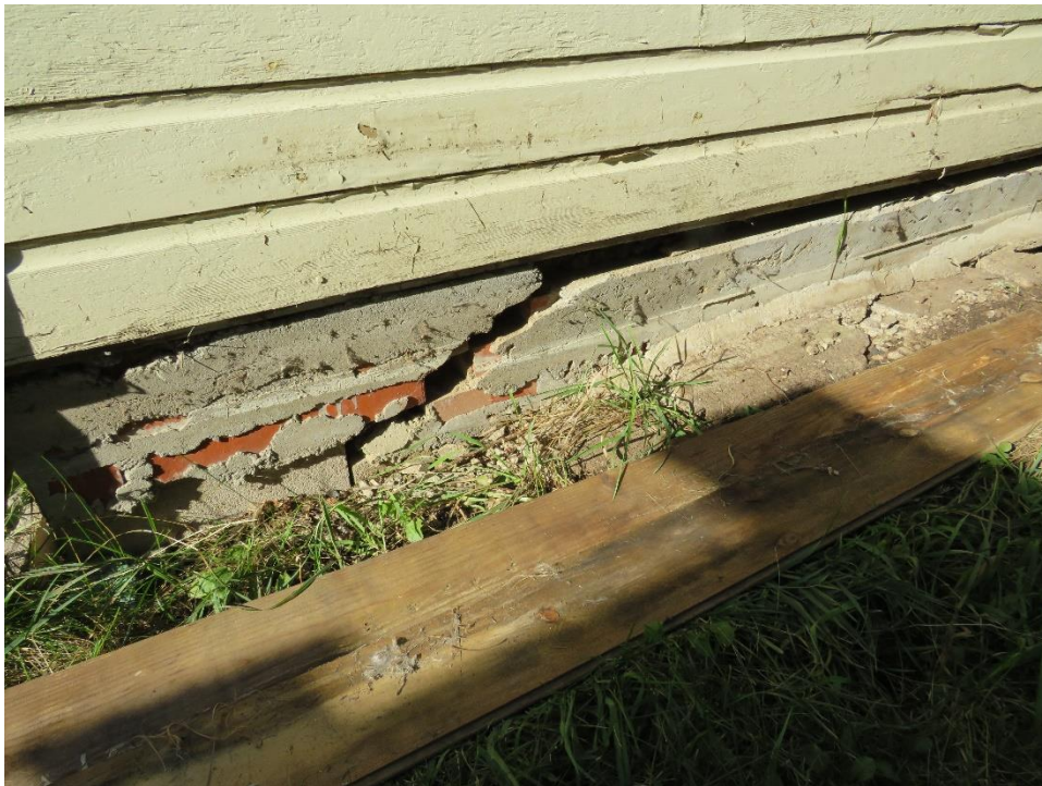
This photograph is the cracked foundation on the left side.
