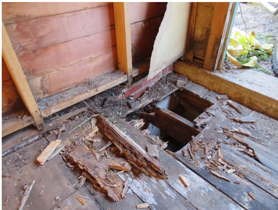
This photograph shows the deterioration of the garage floor and the two separate bottom plates.
