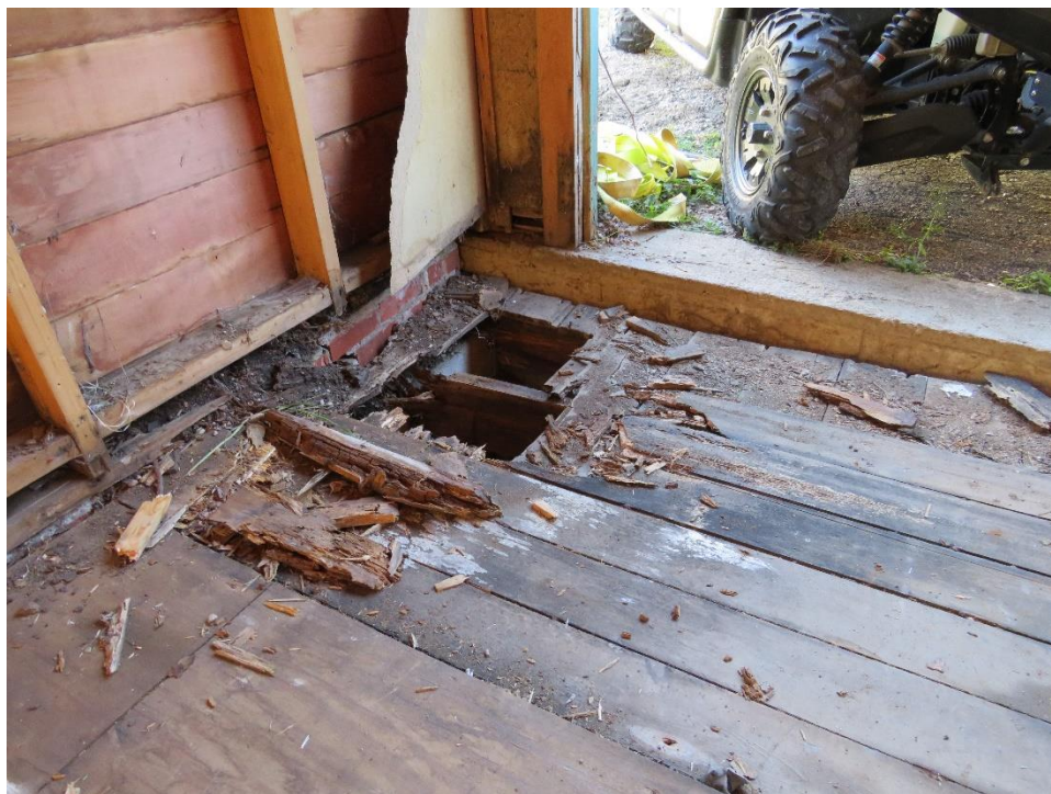
Photograph showing the area of the floor opened up by the applicant verifying construction method and deteriorated conditions.
