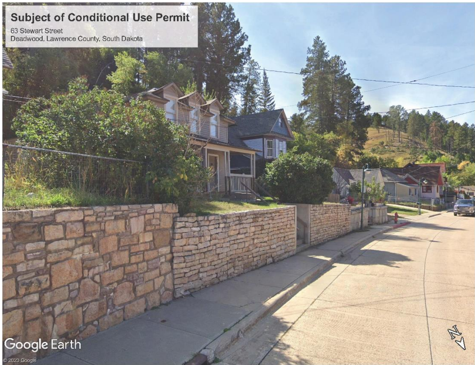
Street view of subject property
