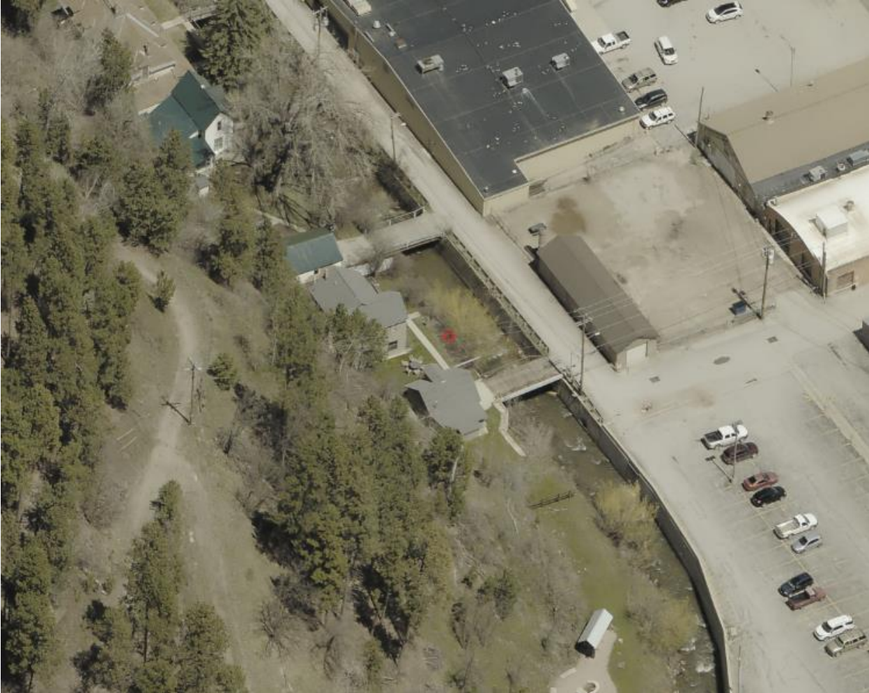
Aerial view of 36 Water Street.
