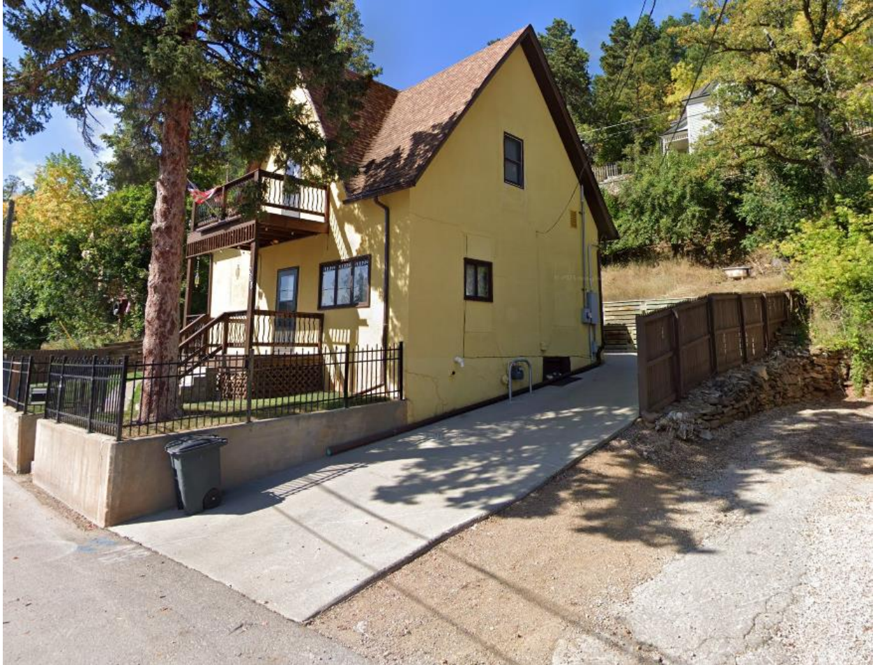
Photo showing proposed location of driveway expansion and new garage at 288 Williams St.
