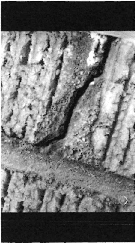
Brick Restoration of brick. Masonry caulked (GREY)
