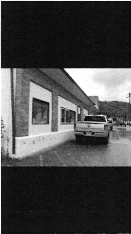
Front of Building
