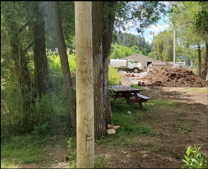
B OVERVIEW OF SITE
