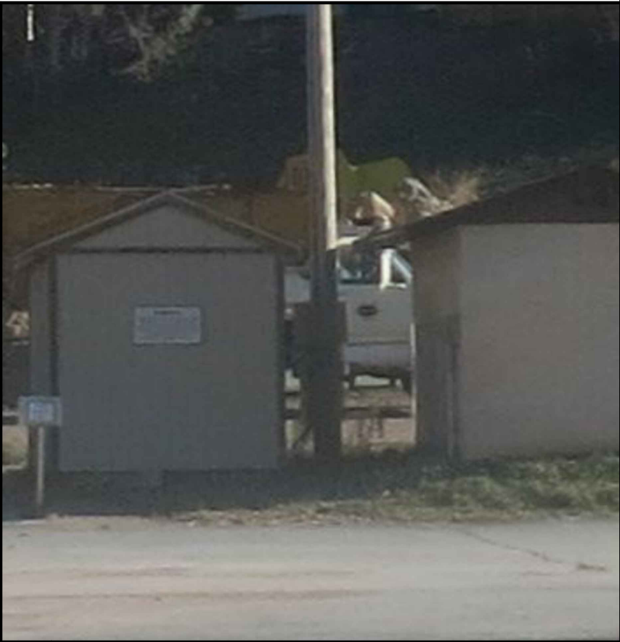
D OVERVIEW OF SITE
