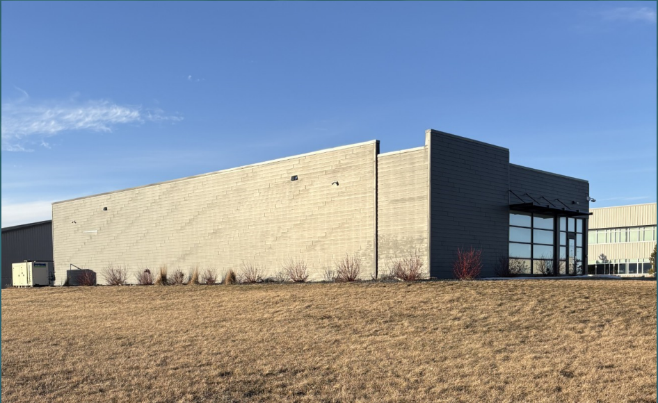
Back and side of building (view from Southeast)
