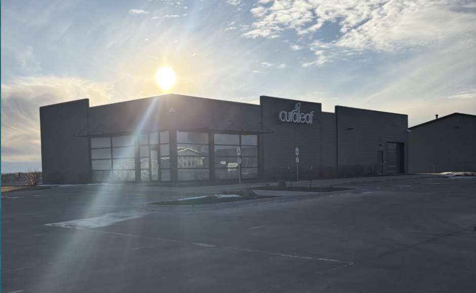
Front of building (view from Northeast)
