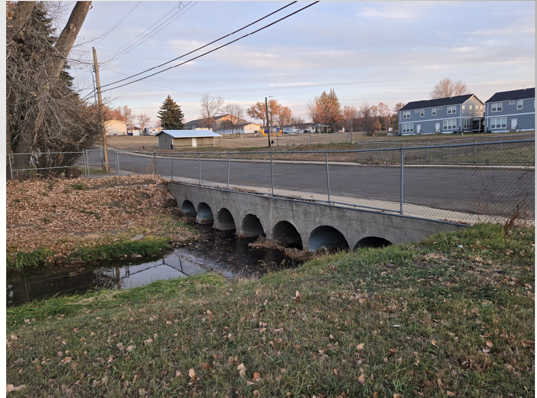
Drainage ditch debris was removal on 8 th Ave. E.
