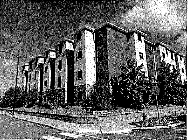
Building elevation facing northwesterly
