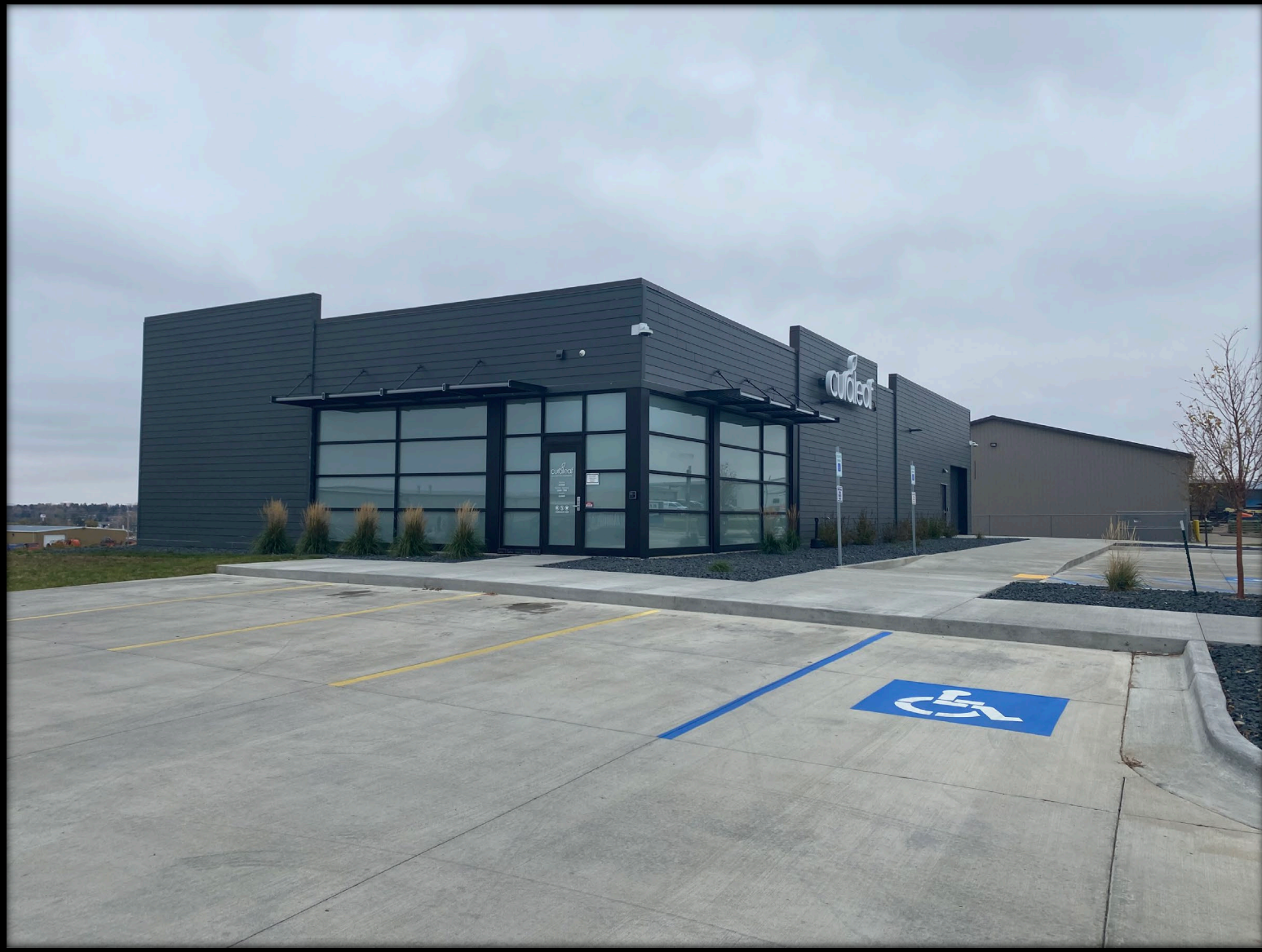
Front of building (view from Northeast)
