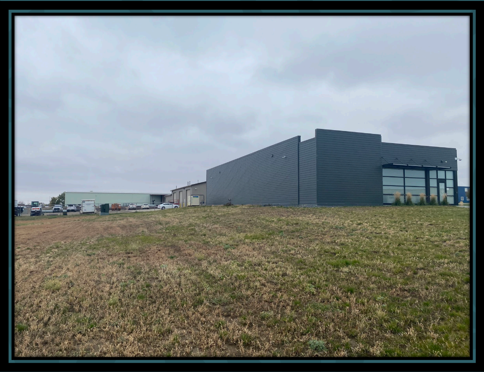
Back and side of building (view from Southeast)
