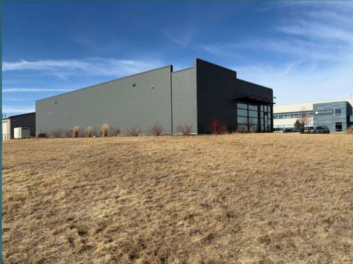
Back and side of building (view from Southeast)
