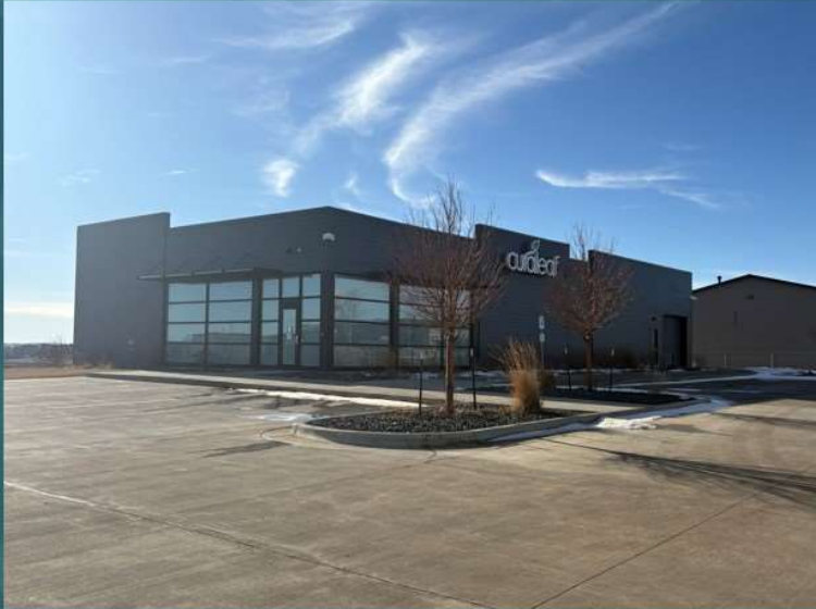
Front of building (view from Northeast)
