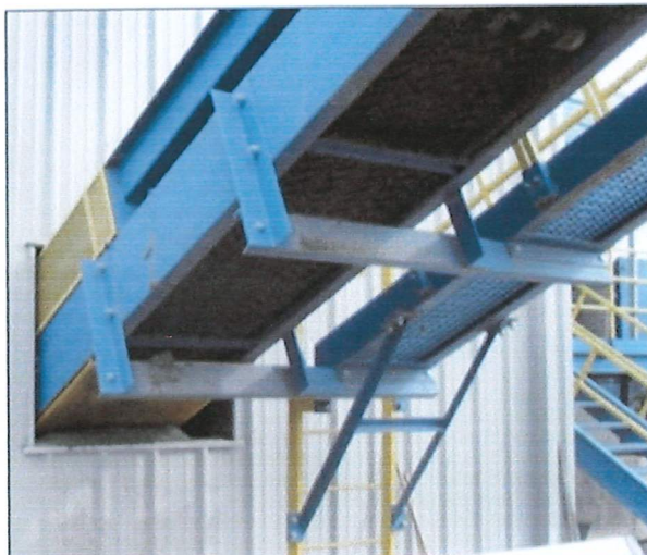
Figure 9. Shredder conveyor opening.
