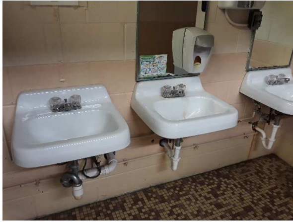
Lavatories – Pool Locker Room
