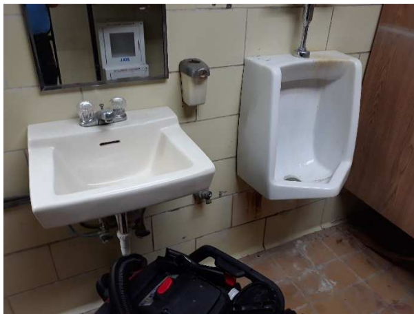
Typical Toilets – Original Building
