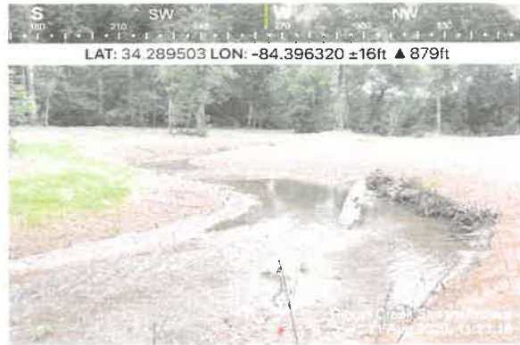
Re-worked stream bankfull dimensions & bench
