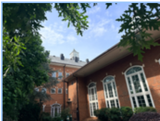
Smoke Evac Fans (Exterior View)
