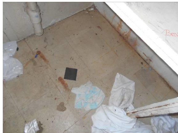
Photo #12 View of the ACM vinyl composite tile (HA-20) in the maintenance area.
