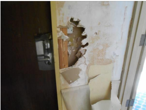
Photo #15 View of the ACM joint compound and textured (HA-25) wall surface in guest room.
