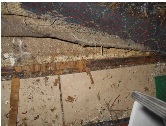
Photo #11 View of the ACM vinyl composite tile (HA-5) under carpet in the lobby area.
