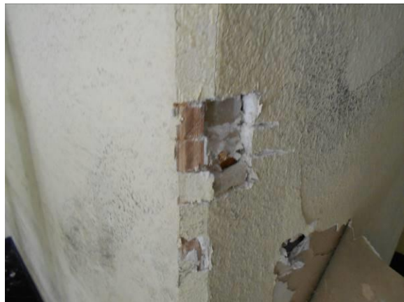
Photo #16 View of the ACM joint compound (HA-26) and textured wall surface in guest rooms.
