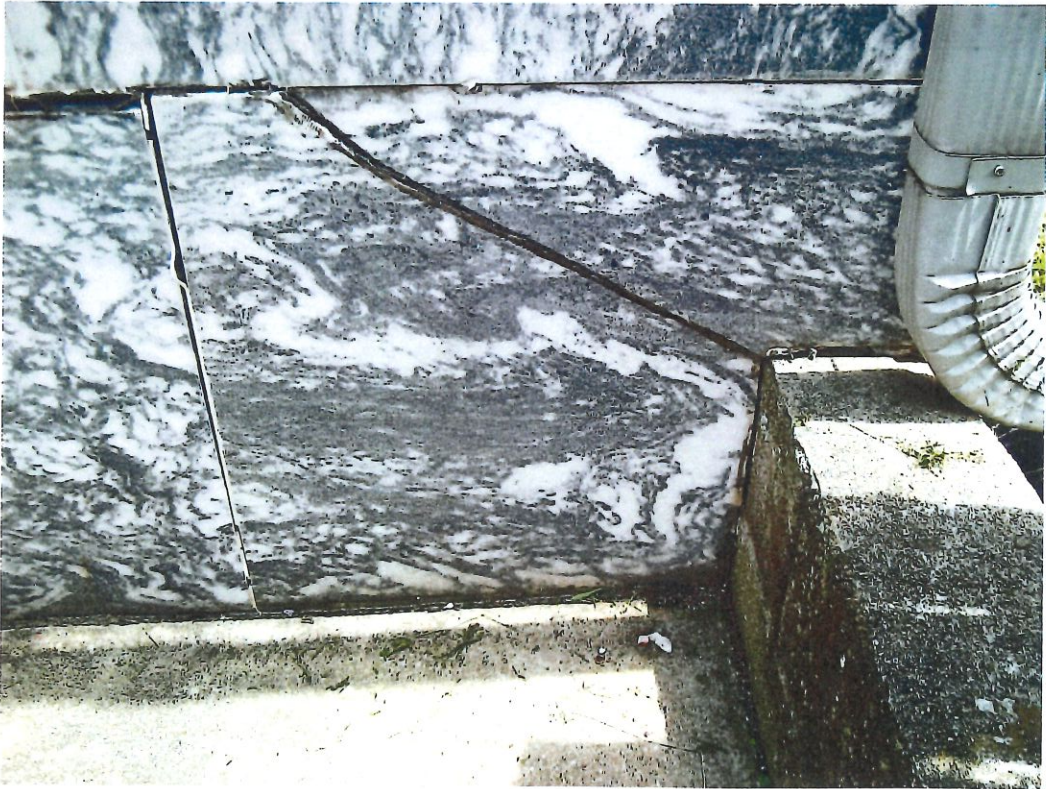
Repair crack in slab and lift sag, re-caulk 1
