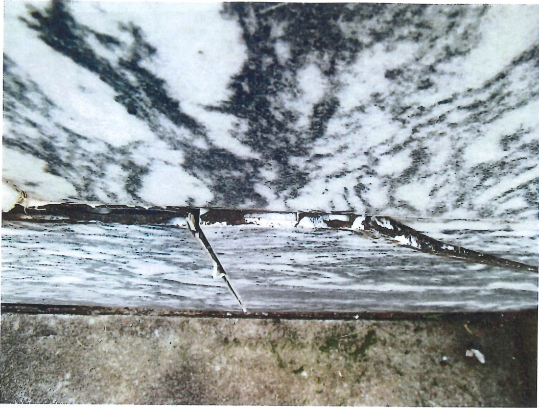
Repair crack in slab and lift sag, re-caulk 2
