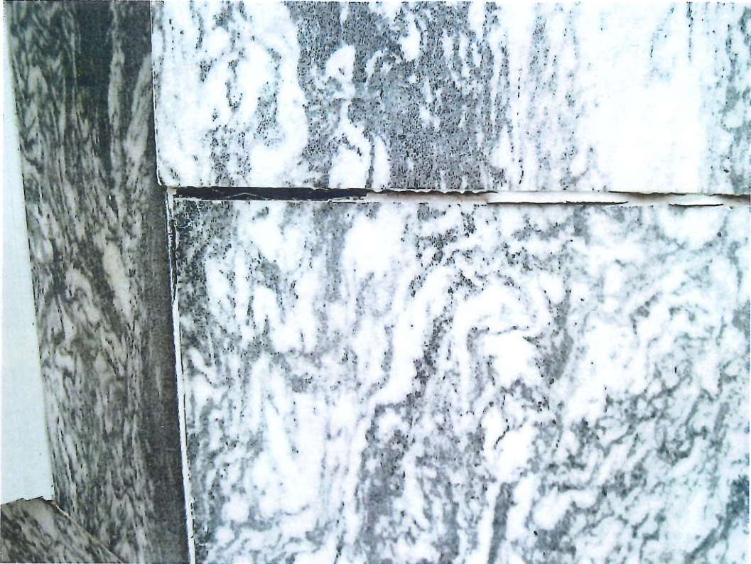
Repair shift, re-caulk
