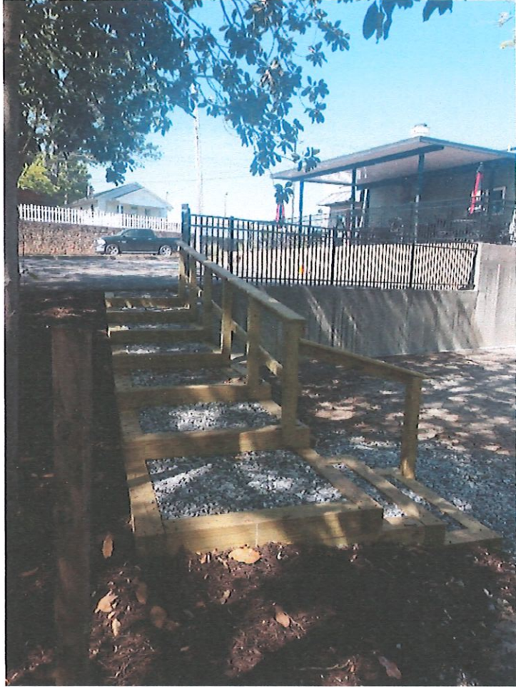
Northerly facing adjacent building/Main Street view
