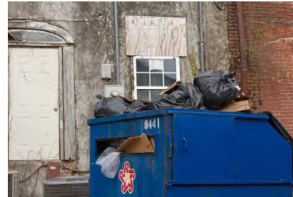
Example of unscreened service area.
