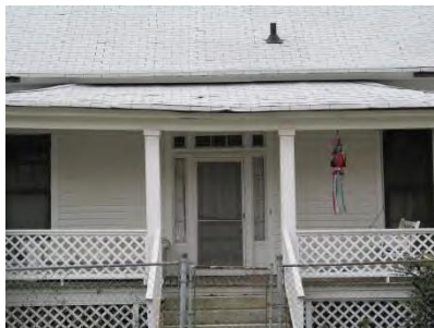
Lattice is inappropriate material for a porch or deck railing.
