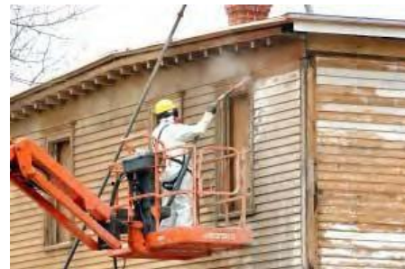
Cleaning wooden features and surfaces with destructive methods such as power washing is inappropriate.
