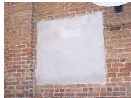
Damaged masonry should be replaced in kind rather than with another material.
