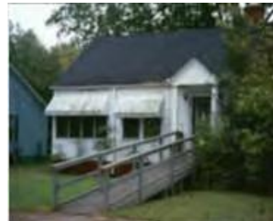
Example of inappropriate placement and lack of screening for handicap access ramp.
