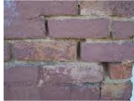
Crumbling Mortar should be repointed.
