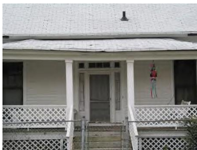
Lattice is inappropriate material for a porch or deck railing.
