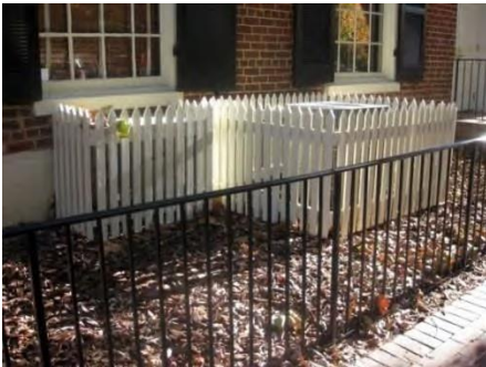
Example of appropriately screened HVAC units.
