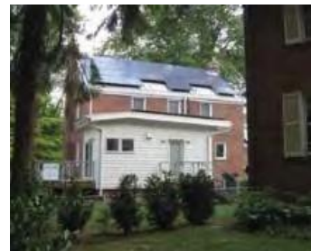
Solar panels have been installed at the rear; however, because the house is situated on a corner, they are highly visible and negatively impact the historic character of the area.
