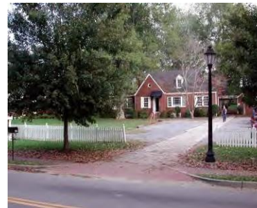
Example of Inappropriate Treatment: Parking constructed in front of main structure and not adequately screened detracts from the historic character of the property.
