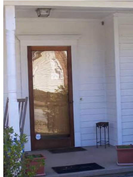
Example of an appropriate entrance way.
