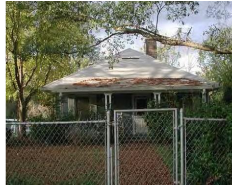
Example of Inappropriate Treatment: Chain-link fence in front yard. Fence is not adequately screened. Height is excessive and obscures view of historic structure.
