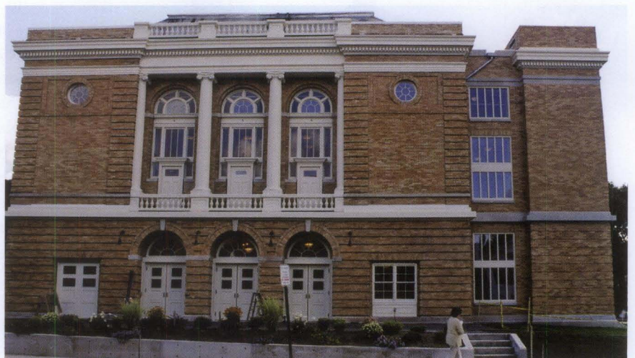
Figure 7. A vacant side lot was the only place a new stair tower could be built when this 1903 theater was rehabilitated as a performing arts center. Constructed with matching materials, the stair tower is set back with a recessed connector and, despite its location, it is clearly subordinate and differentiated from the historic theater.
