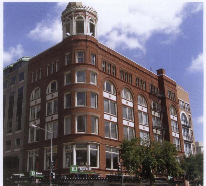
Figure 30. The small addition on the right of this late-19th century commercial structure is clearly secondary and compatible materials and design with the historic building.
