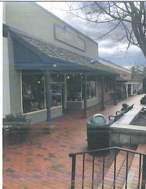
Pic. 5 Columns - General Store
