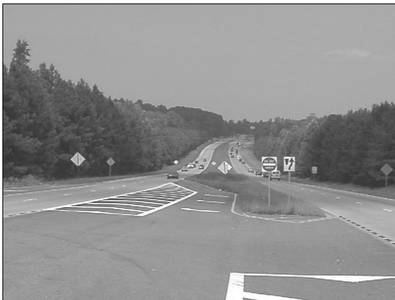
GA 400 North, north of commercial center at intersection of SR 53
