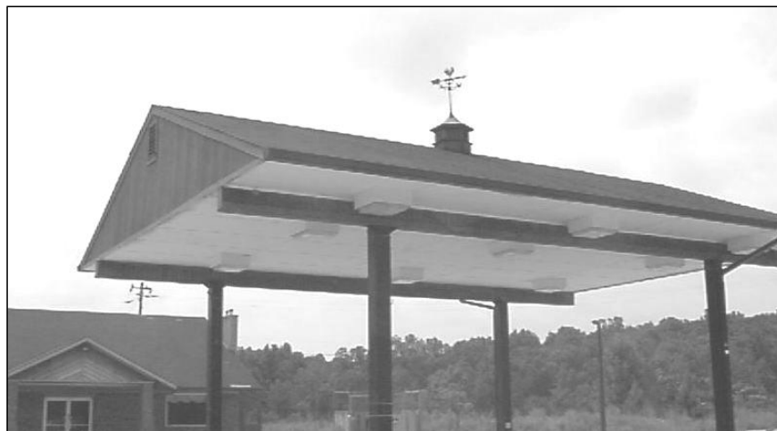
Shopping center northbound on Ga. 400 north of SR 136
