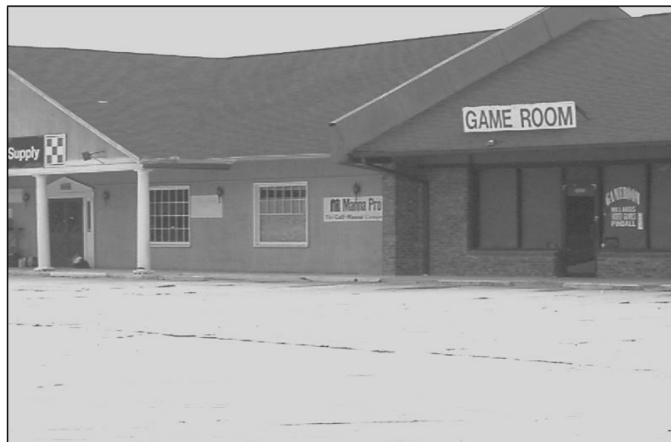
Shopping center northbound on Ga. 400 north of SR 136
