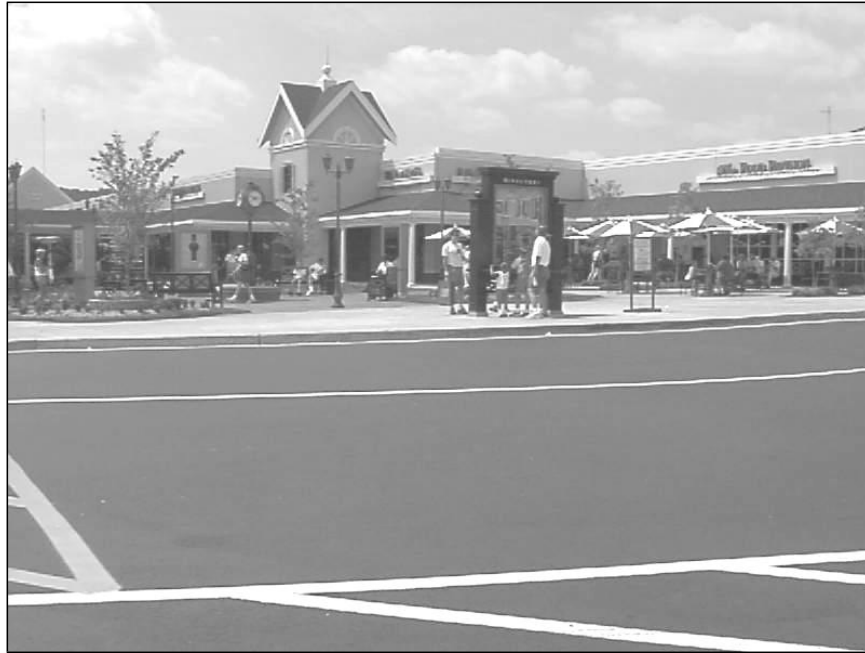
Public Space and Pedestrian Amenities at North Georgia Premium Outlets
