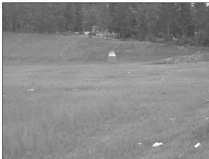
Graded site adjacent to Kroger Shopping Center
