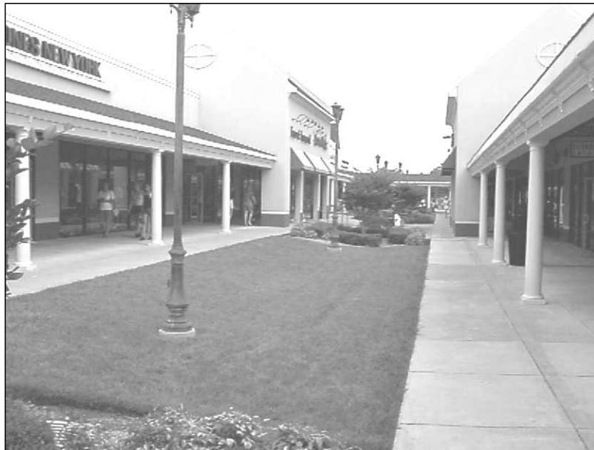
Pedestrian Corridor at North Georgia Premium Outlets
