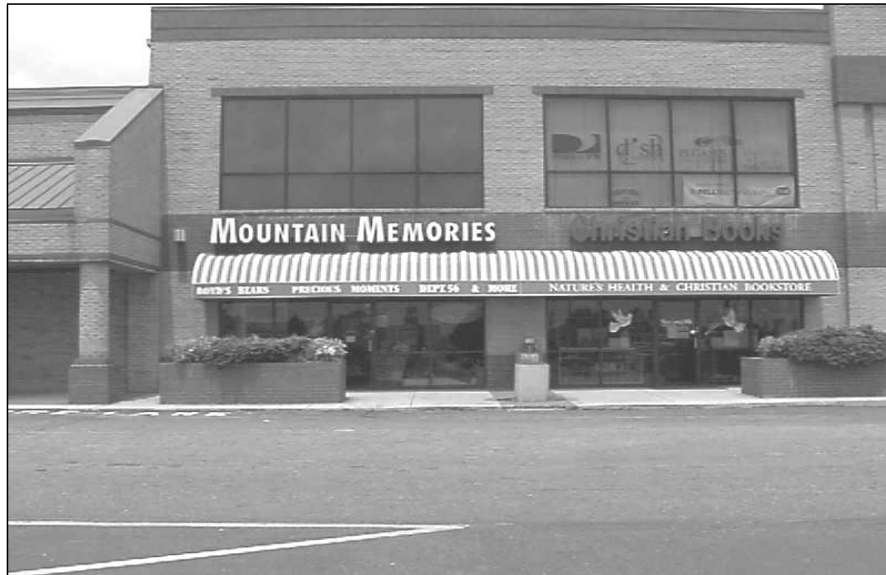
Dawson 400 shopping center at Ga. 400 and SR 53 (southwest quadrant)
