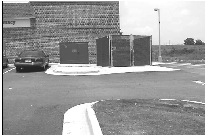
CVS pharmacy on north side of SR 53 west of Ga. 400
