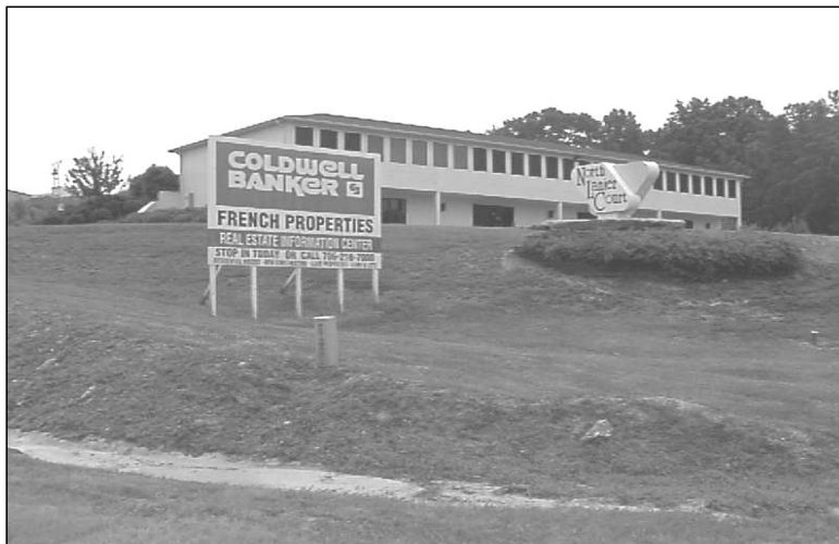
North Lanier Court, Ga. 400 northbound of SR 53
