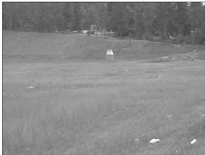
Graded site adjacent to Kroger Shopping Center
