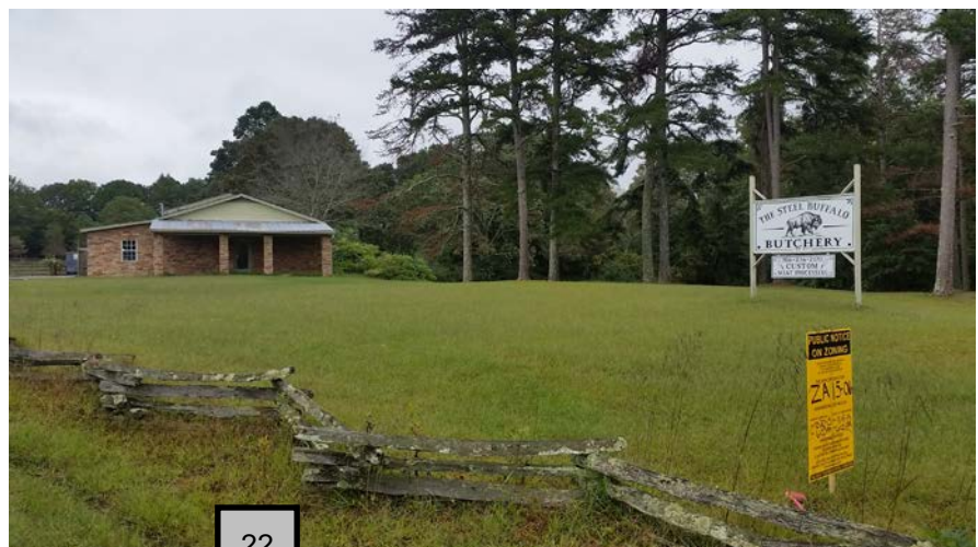
Existing commercial building on subject property.
