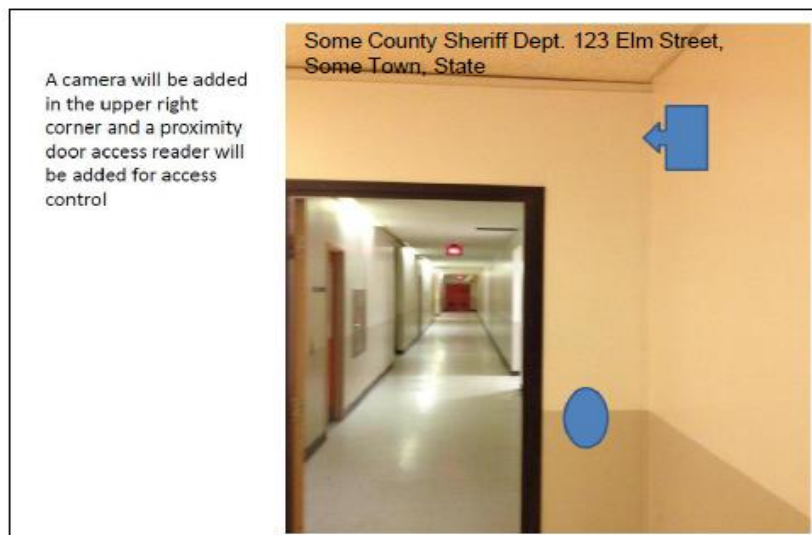
Figure 6. Interior photograph showing proposed location of new equipment.
