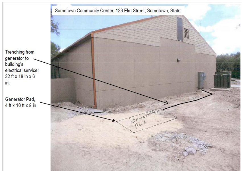
Figure 4. Ground-level photograph showing proposed ground disturbance area.
