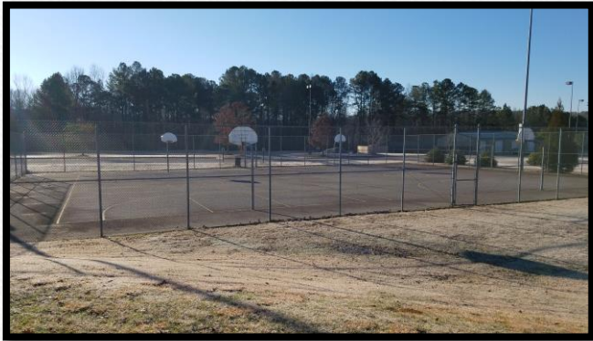
Existing Basketball Courts
