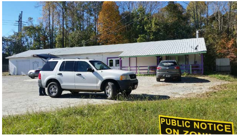
Existing commercial building on subject property.
