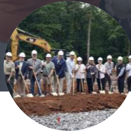
Groundbreaking for Amicalola's Visitor's Center
