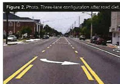
Figure 2. Photo. Three-lane configuration after road diet.
