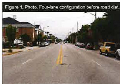
Figure 1. Photo. Four-lane configuration before road diet.
