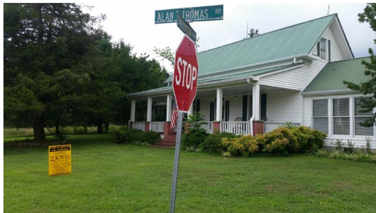
Subject property existing residence to be used for proposed business
