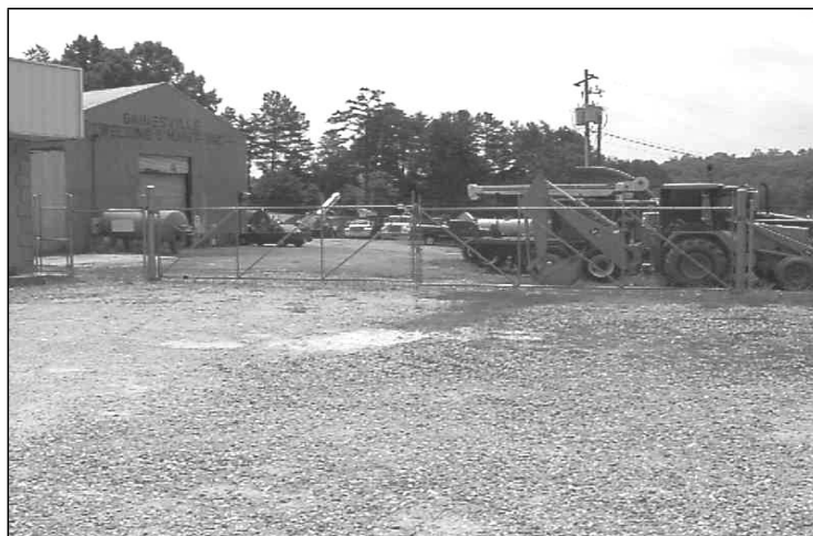
Gainesville Welding and Maintenance, Henry Grady Highway
