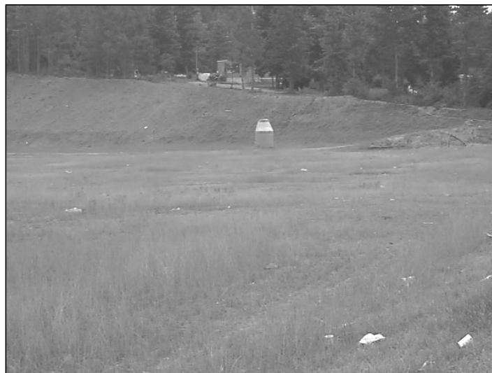
Graded site adjacent to Kroger Shopping Center
