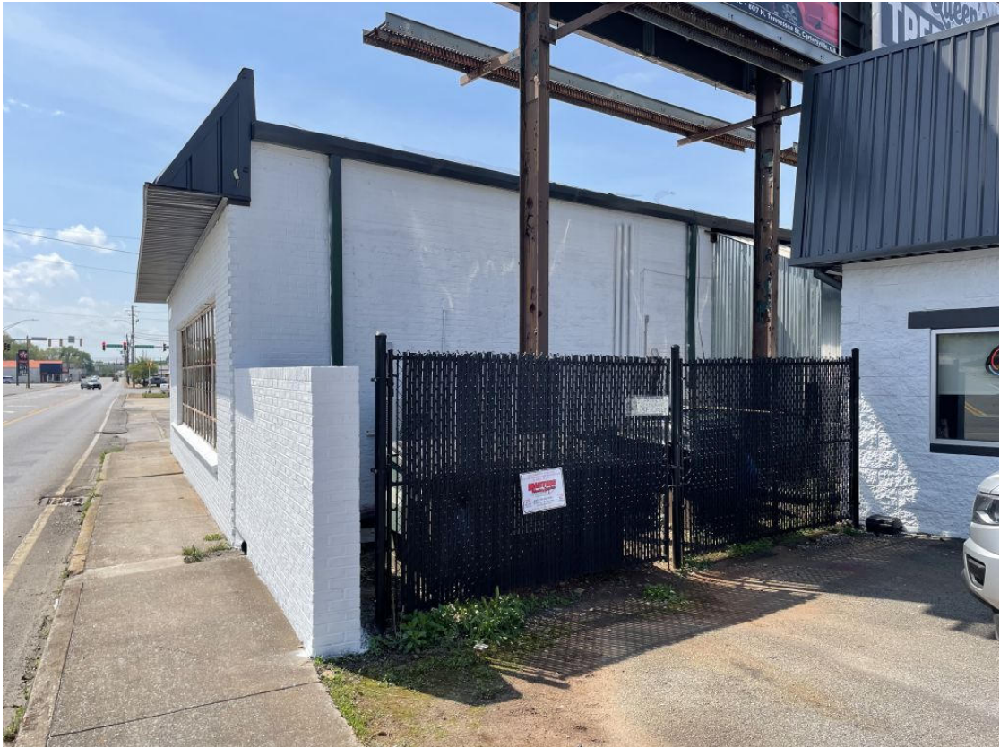
Rear of 120 Building and side wall of 117 Building from Tennessee St.
