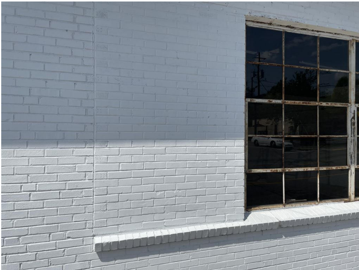
Tennessee St side. Window Opening bricked-in.
