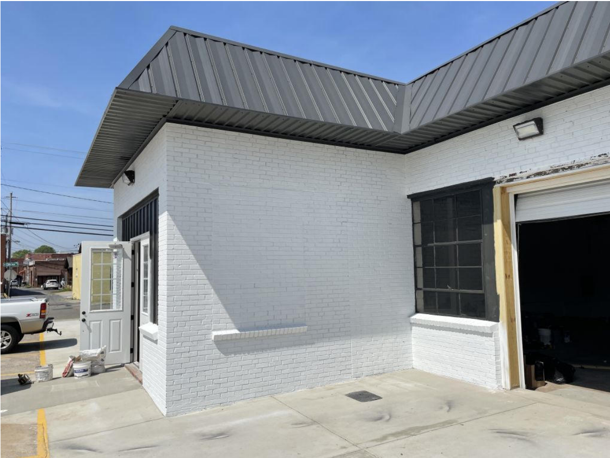
Window and standard door openings bricked-in.
