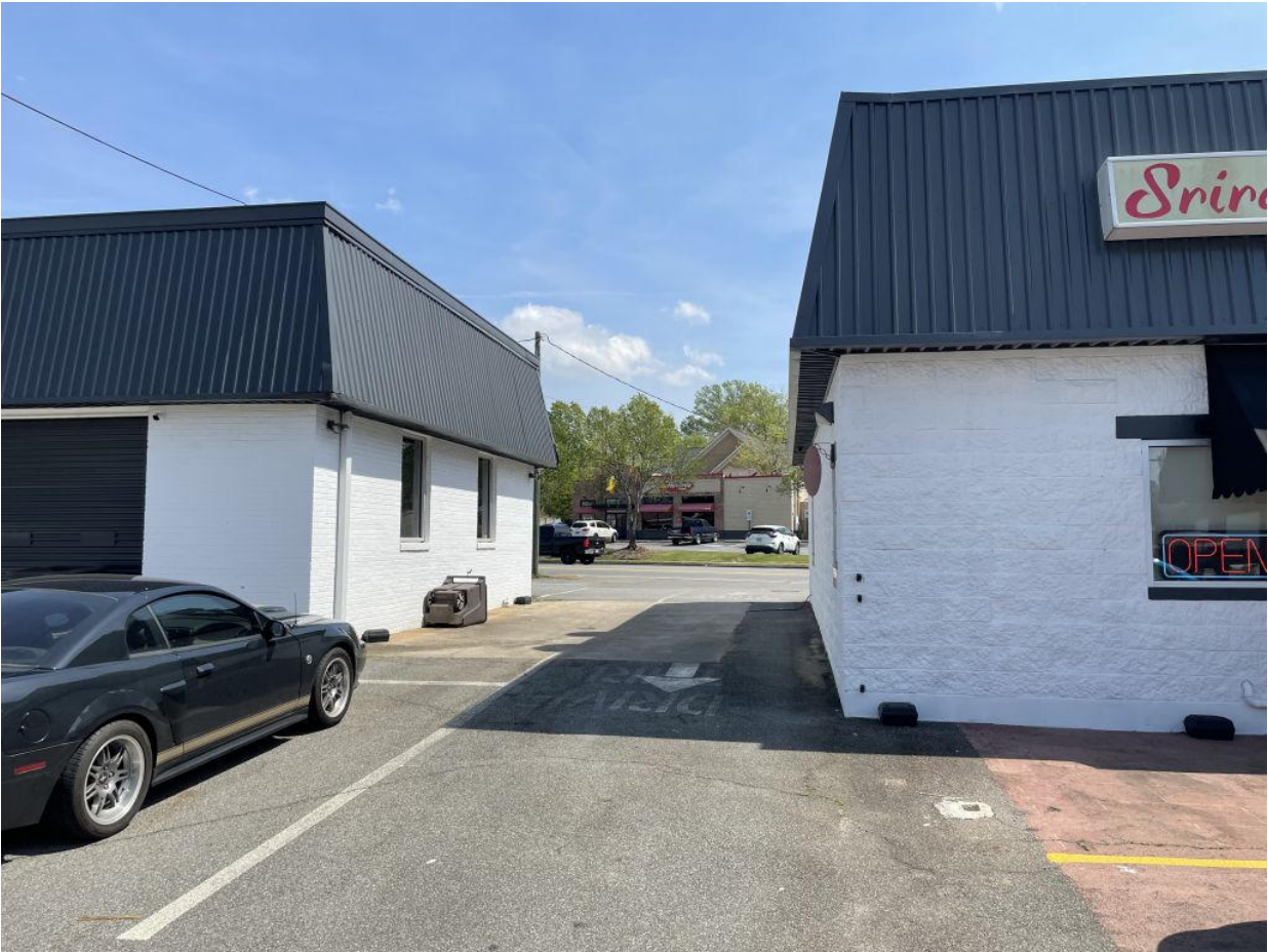
103 and 117 Building from Gilmer St.
