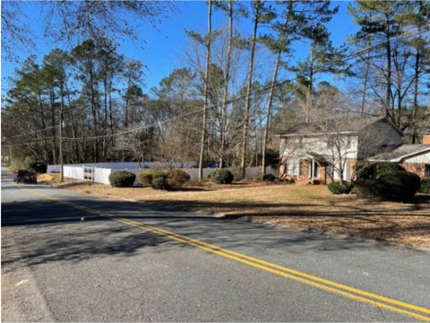
Current view of back of 108 Mitchell Ave. with fence on Plymouth Dr.
