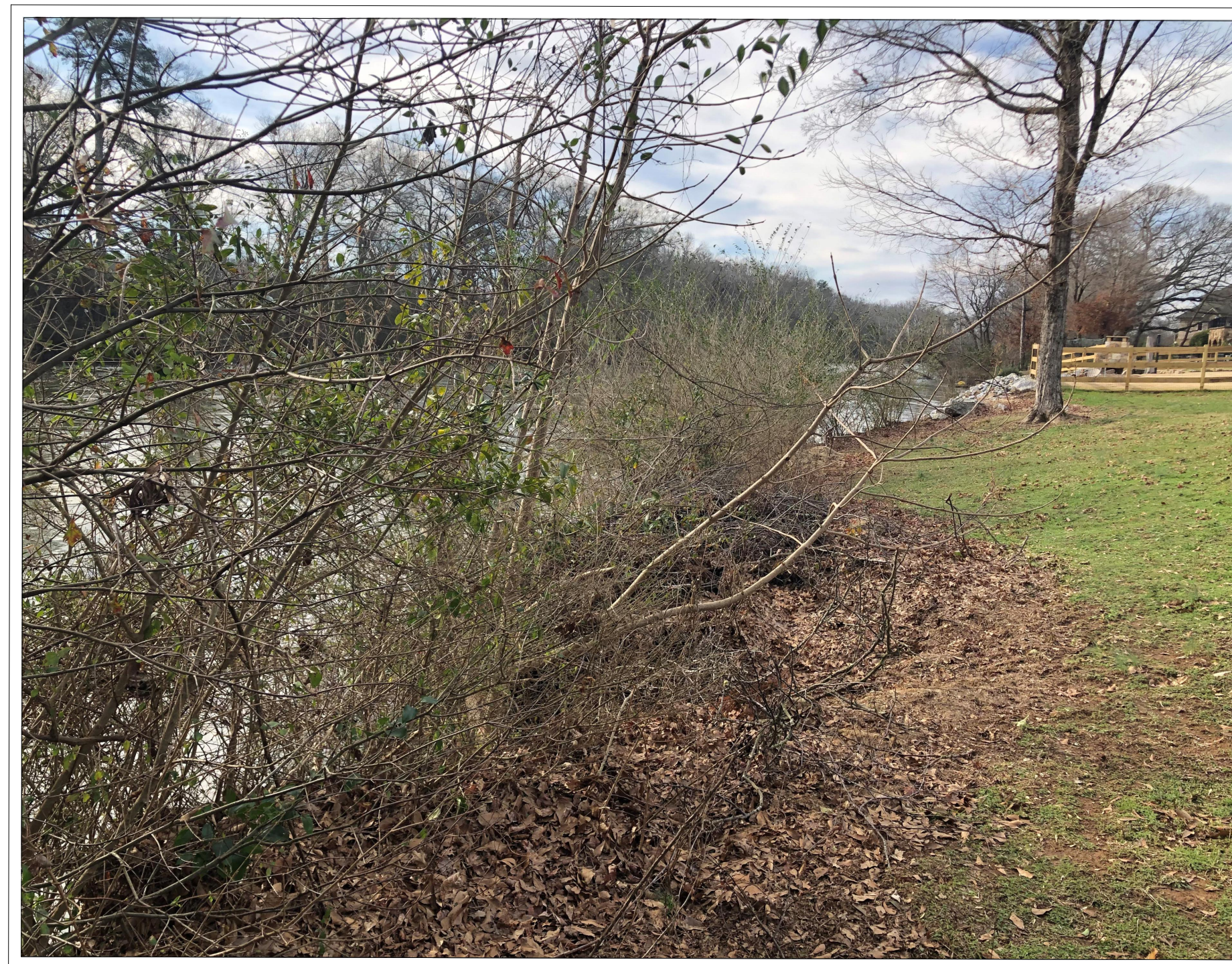
PICTURE "2" RIVER BANK ERODING
