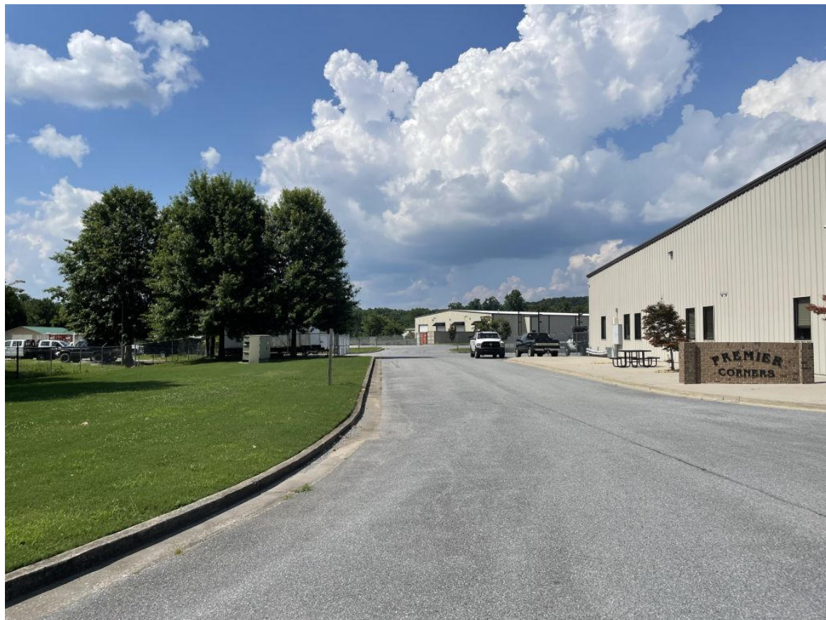
View from Curtis Ct along left side of Building 30. Building 44 is in the distance.
